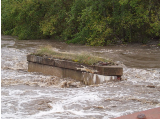
A bridge pier at the "Old Highway 61" in Kellogg. Located just downstream of the stabilization project this picture was taken very close to the river crest.
