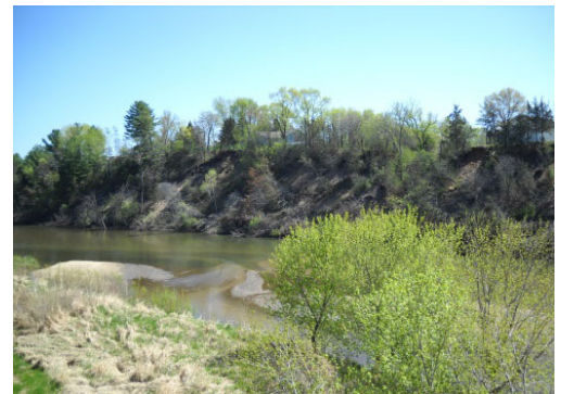
This image shows part of the failing stream bank. Mature trees gave way and you can see homes just behind the tree line above the bank.
