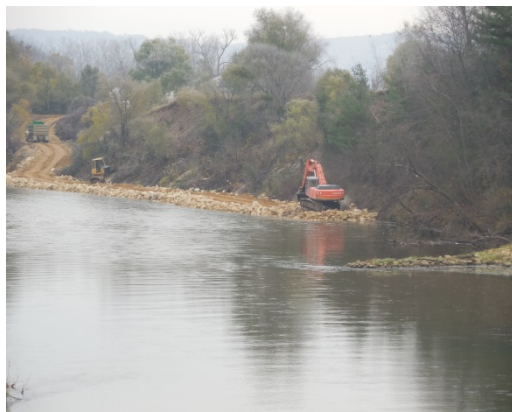
Construction of Phase 2 which worked upstream and connected to the downstream end of Phase 1.
