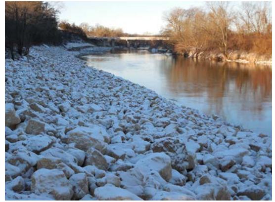
All phases of construction were completed in November of 2013, just before the first snowfall of the year.
