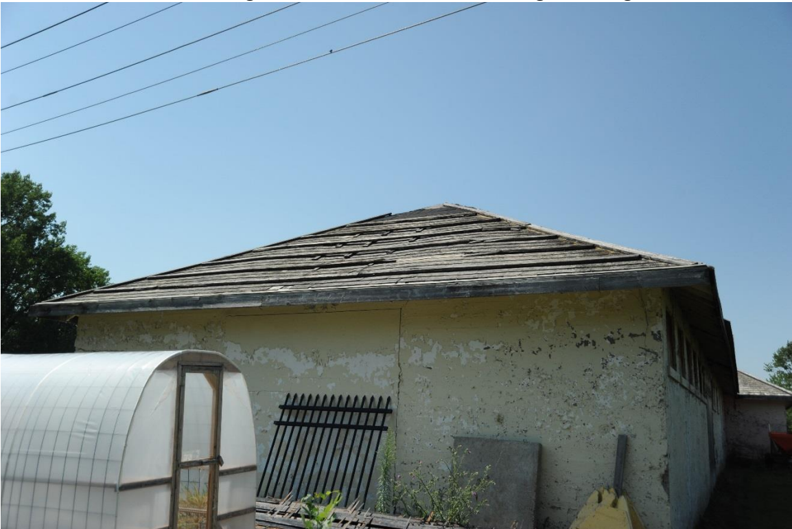
1. AP: Fergus Falls: walls and roof on storage building
