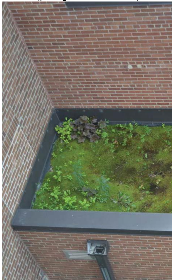
1. AP: Minneapolis: roof replacement and repair (plant growth not desired)
