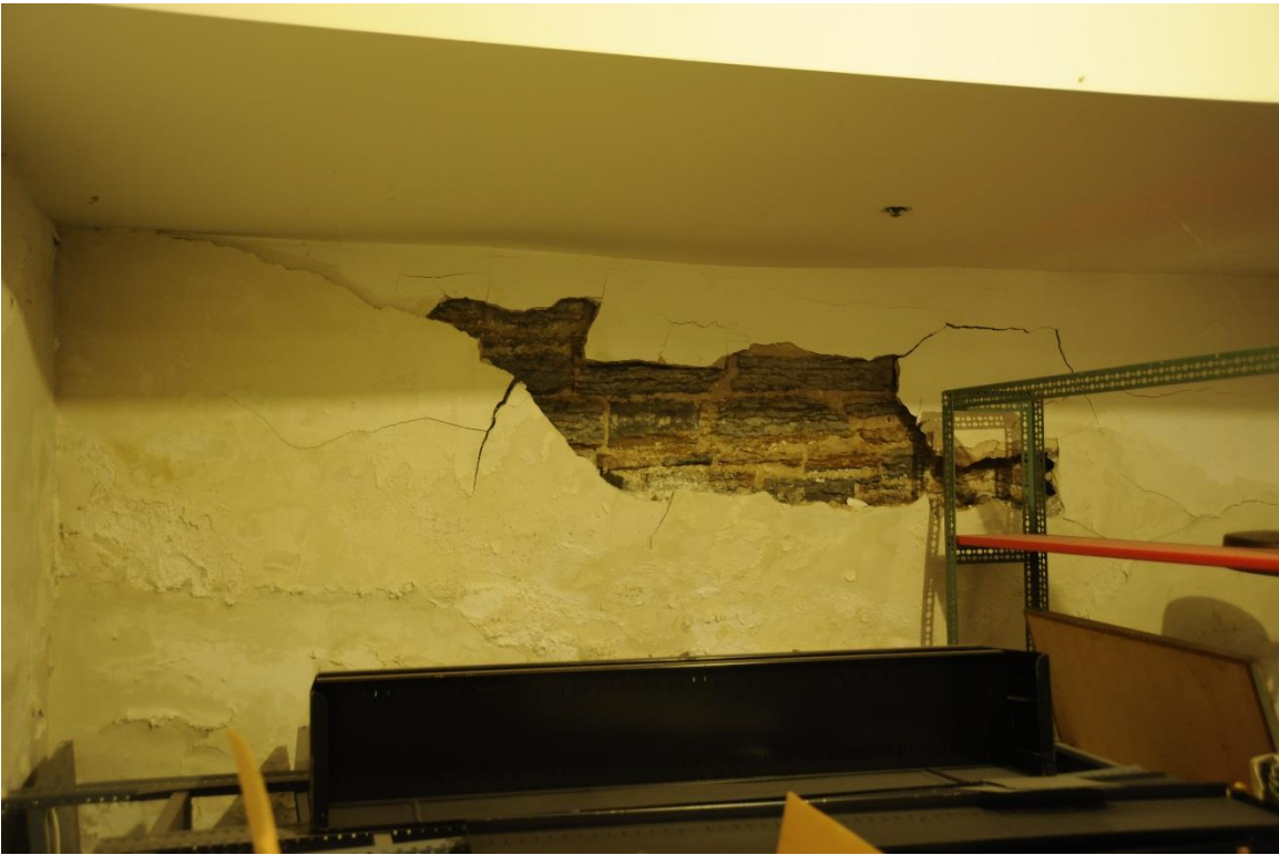
1. AP: Minneapolis: foundation wall repair
