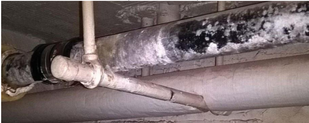
1. AP: Minneapolis: water line replacement
