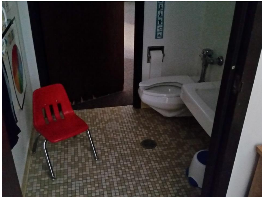
Quinn Hall: Outdate inaccessible bathroom
