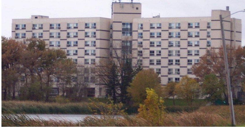
Lakeview Highrise, Willmar Preservation project to replace plumbing Publicly owned by Kandiyohi County Housing and Redevelopment Authority, 121 units
