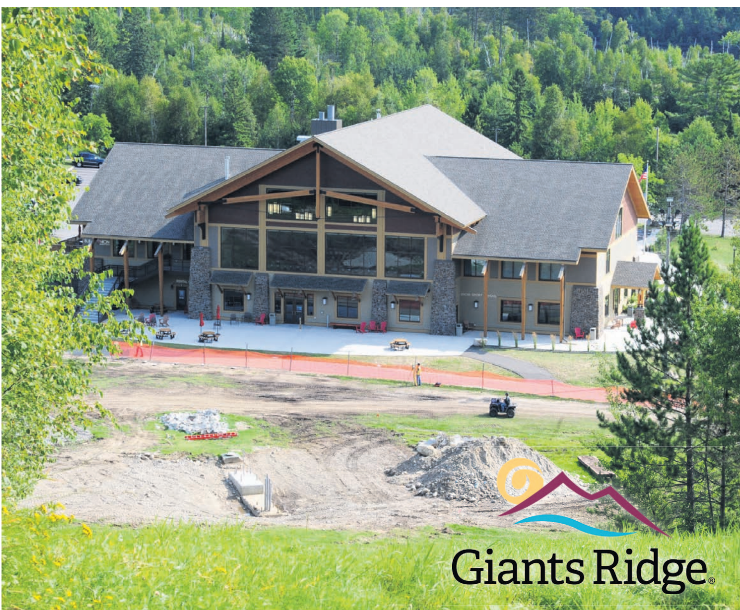
Construction is beginning on two new ski lifts at Giants Ridge.
