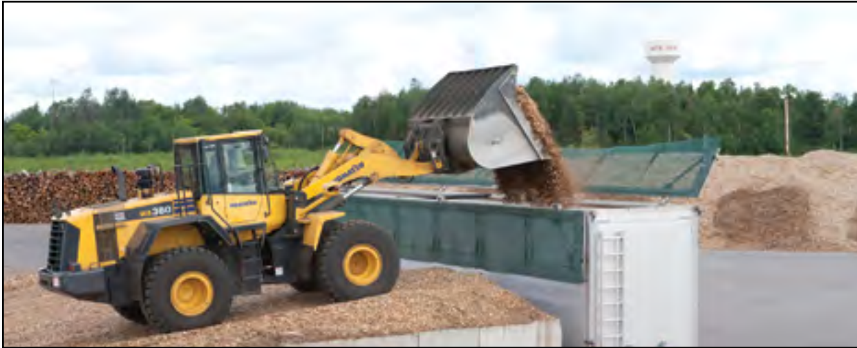
The agency financially supported the construction of the Laurentian Energy biomass boiler project at Virginia Public Utilities and Hibbing Public Utilities.
