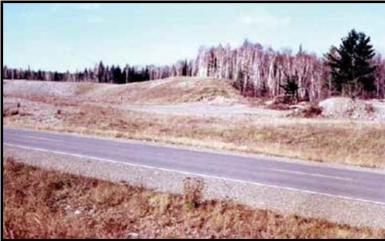
Rehabilitate gravel pits upon completion of use. Photo courtesy of Superior National Forest
