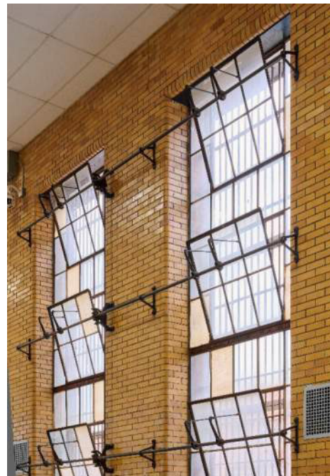
Image 2: Original windows in dining hall. Photo by Ryan Siemers, 2026.
