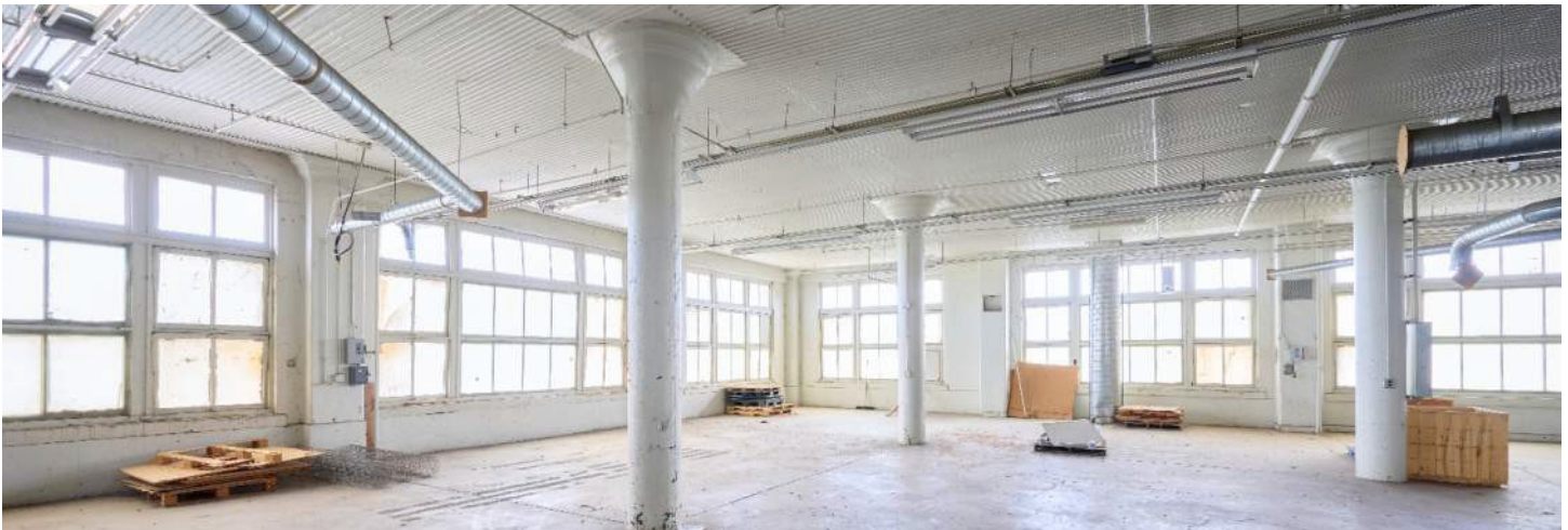
Image 12: Interior of Building 21. Photo by Ryan Siemers, 2026.
