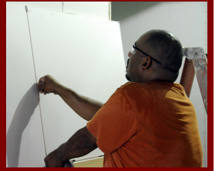
An offender in the ICWC Program hangs sheetrock
