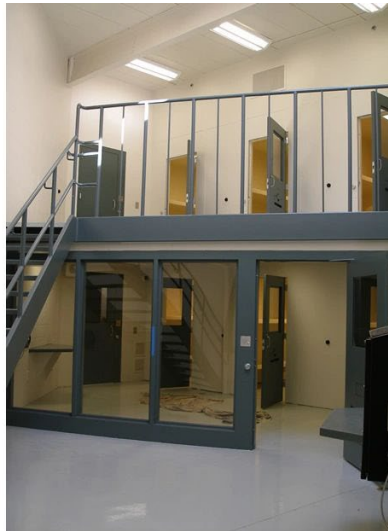
Figure 4. Example of a mezzanine 151
