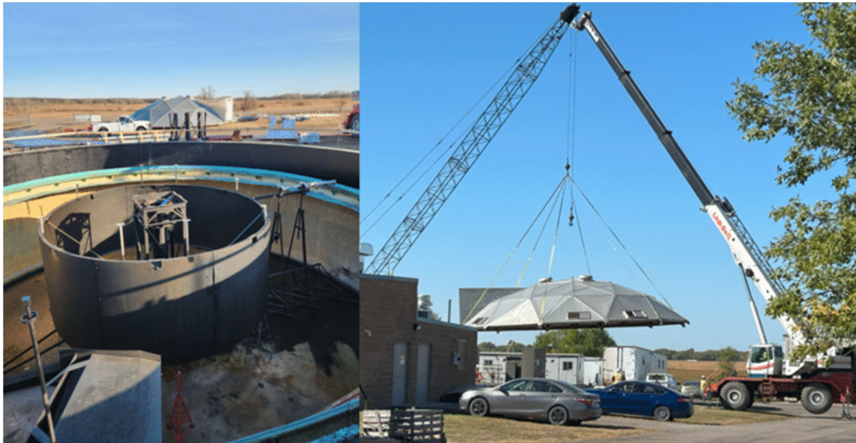
Kandiyohi County: GLSSWD Wastewater Treatment Facility Improvement Project
