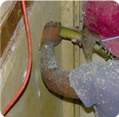
7. Dense pack stairway walls
