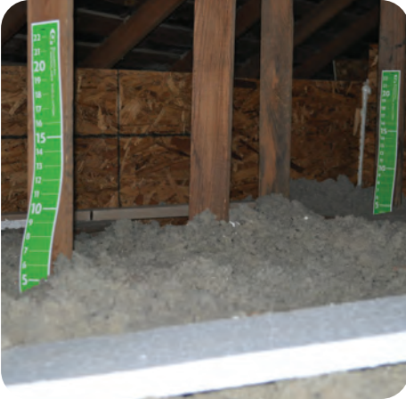
5. Depth rulers installed, 1 per 300 square feet
