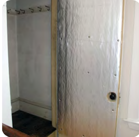
8. Weatherstrip and insulate door
