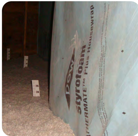
4. Install backing material
