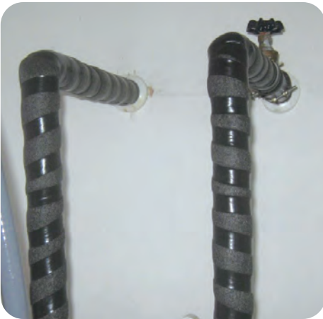
Secure seams with tape
