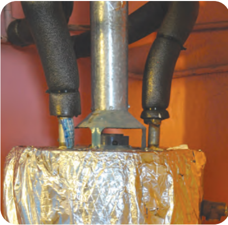
Insulation not kept back at least 6 inches from draft diverter is a fire hazard
