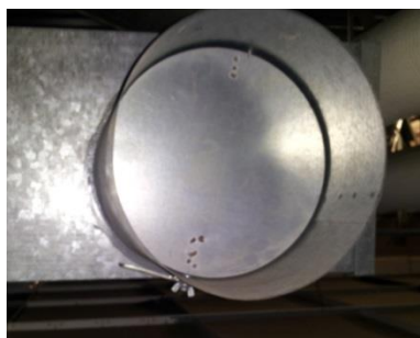
Figure 38: Example of major leakage path discovered via duct inspection: uncapped supply branch sealed with damper only.
