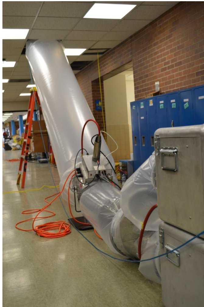
Figure 42: AeroSeal equipment for pressurization testing and sealant delivery setup and ready
