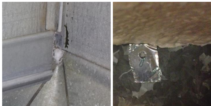
Figure 2: AeroSeal sealant accumulates at the small, distributed leaks in a duct system. The left image shows a large 3/8" corner leak filled with sealant (viewed from inside). The right image shows a 1/4" test hole filled with sealant (viewed from outside)
