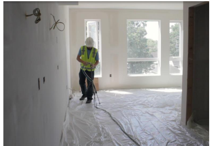
Figure E3. Image of air sealing process in the field
