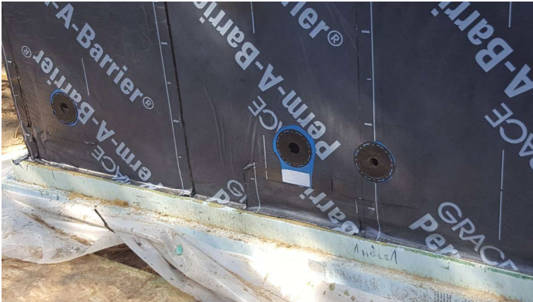
Figure 29 - Example of Prefabricated Flashing
