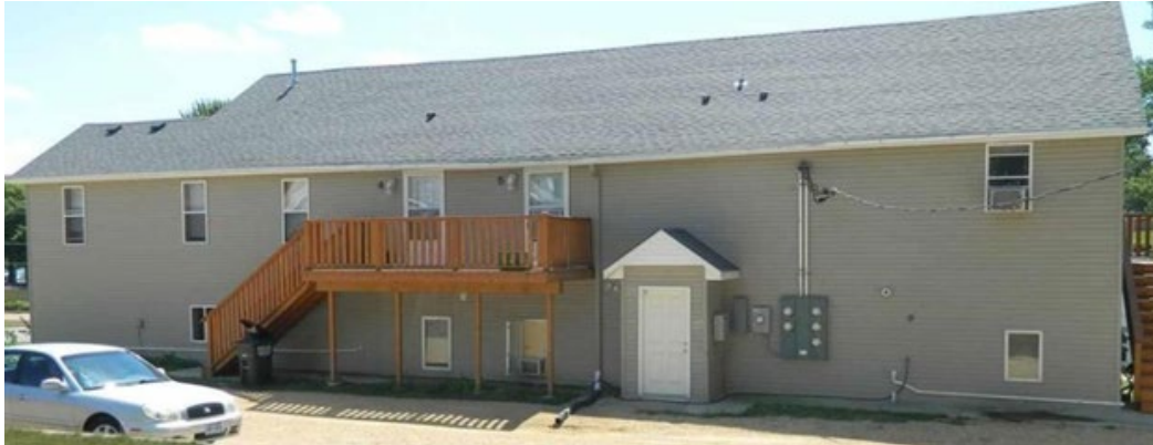
Figure 15 - Example of Temporary Removal for Retrofit
