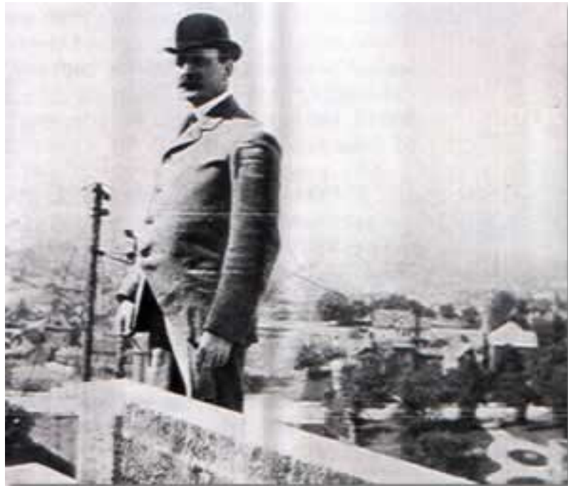
Cass Gilbert standing on the partially constructed state capitol building in Saint Paul, May 9, 1901.
