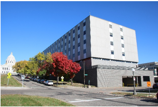
289 290 Image: The Centennial Building on Cedar Street. The Centennial Building on the eastern Mall was built prior to establishment of the 291 CAAPB. Although the Centennial Building meets height, massing and siting requirements, it does not meet expectations of aesthetics 292 appropriate to the architectural integrity sought in government buildings on the Mall. While the design of the Centennial Building was 293 consistent with standard building practices of the day, it prompted the legislature to evaluate the architectural standards for buildings in 294 close proximity to the Capitol. It was in response to this building and others like it developed in the 1950s and 1960s that prompted the 295 establishment of the CAAPB.
