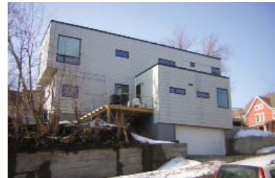
E. Garage access from side street
