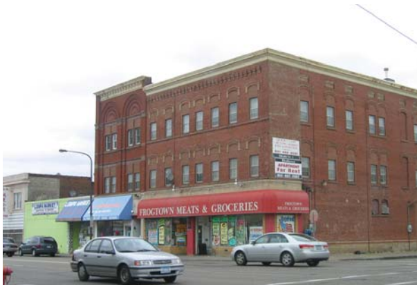
Examples of Typical Buildings in the MX District
