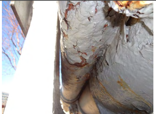
Detail of underside of the PR recoil tube showing condition of metal and paint layers.
