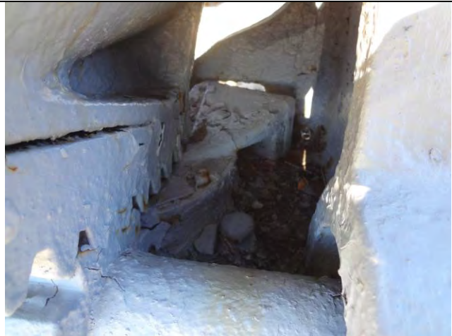
Detail of PL side swivel area showing rust staining.
