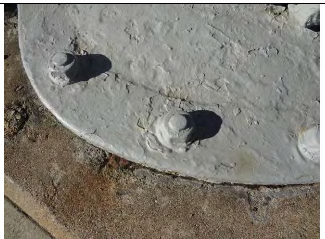
Detail of bolts in base and concrete interface
