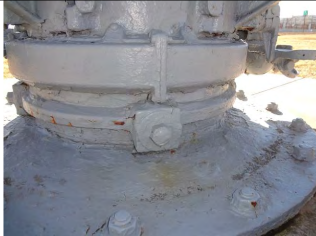
Detail of lower swivel support assembly condition.
