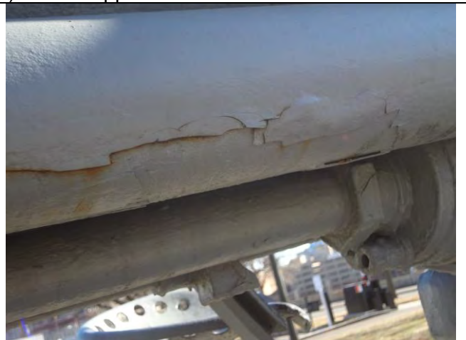
Painting flaking and rust staining on PR recoil tube.
