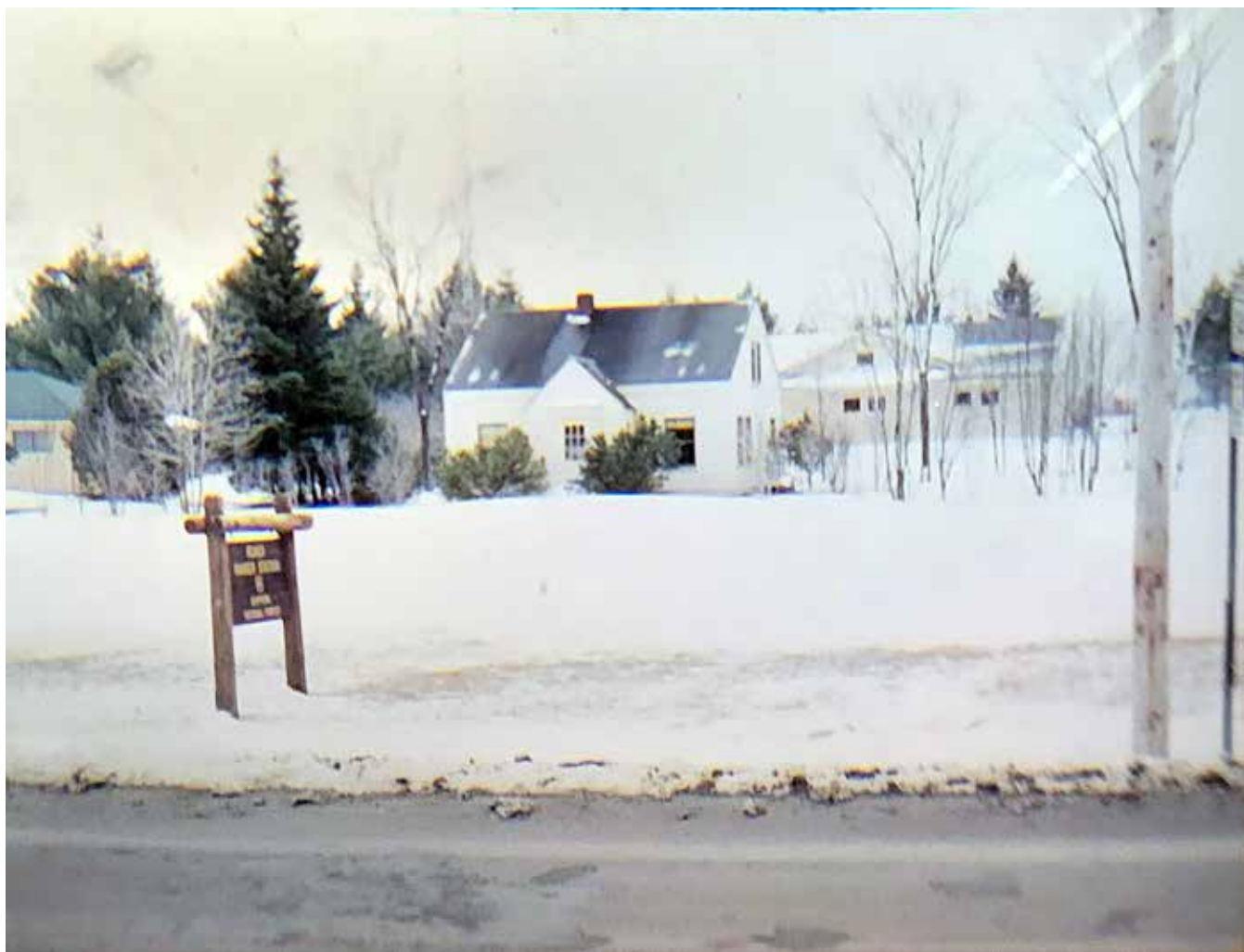
Figure 8: Remer District Ranger Station, Office and Warehouse, 1961. Source: Private Collection
