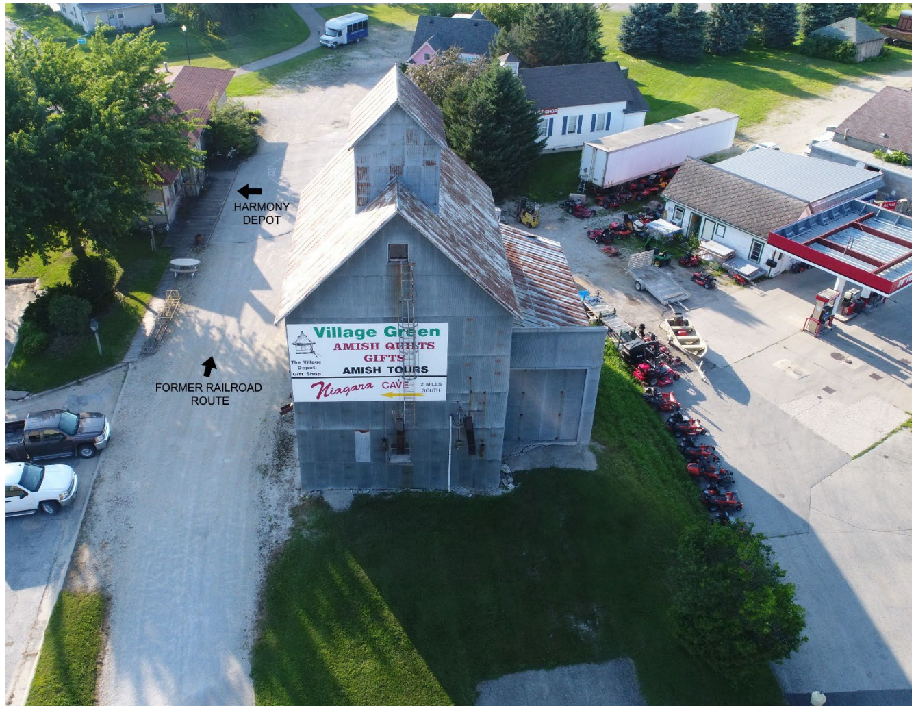
Photo #1 (MN_Fillmore County_Mc Michael Grain Elevator_0001) Overview of historic property and setting. Aerial southeast view.
