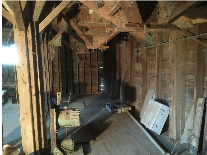
Photo #9 (MN_Fillmore County_Mc Michael Grain Elevator_0009) Interior view of working house floor; west extension with three additional grain bins.
