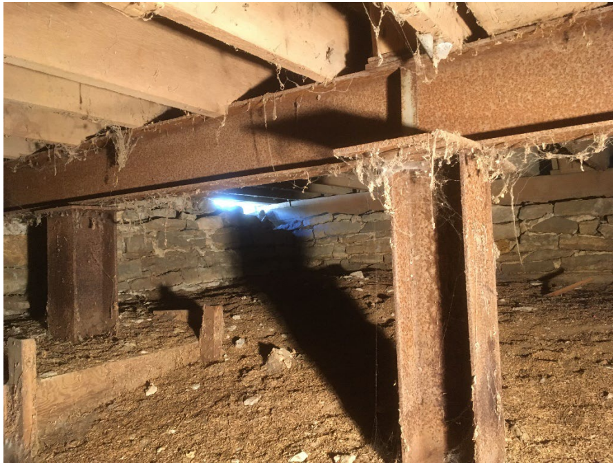
Photo #11 (MN_Fillmore County_Mc Michael Grain Elevator_00011) I – Beam support.
