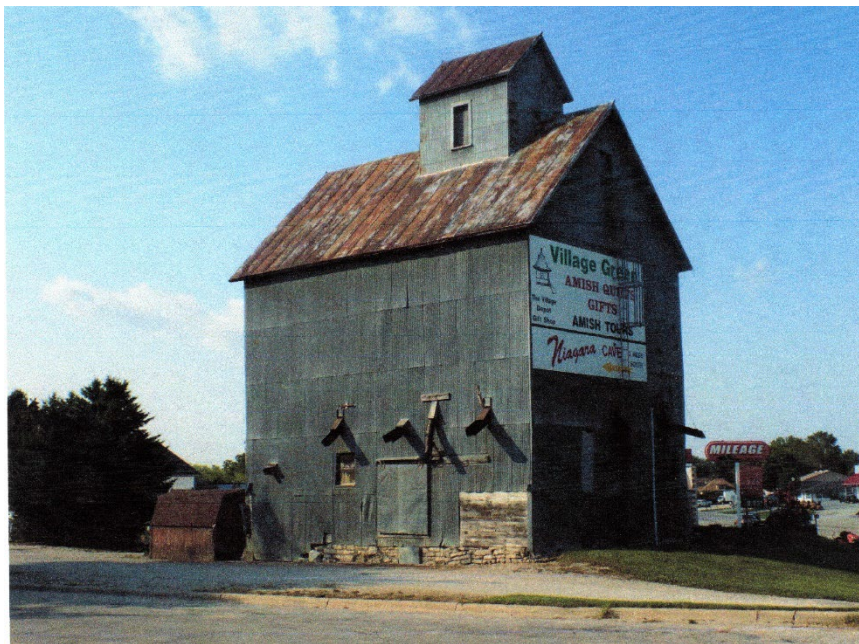
Photo #3 (MN_Fillmore County_Mc Michael Grain Elevator_0003) View of south elevation. Facing northwest.
