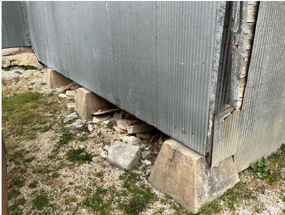
Photo #13 (MN_Fillmore County_Mc Michael Grain Elevator_00013) Addition pier support.
