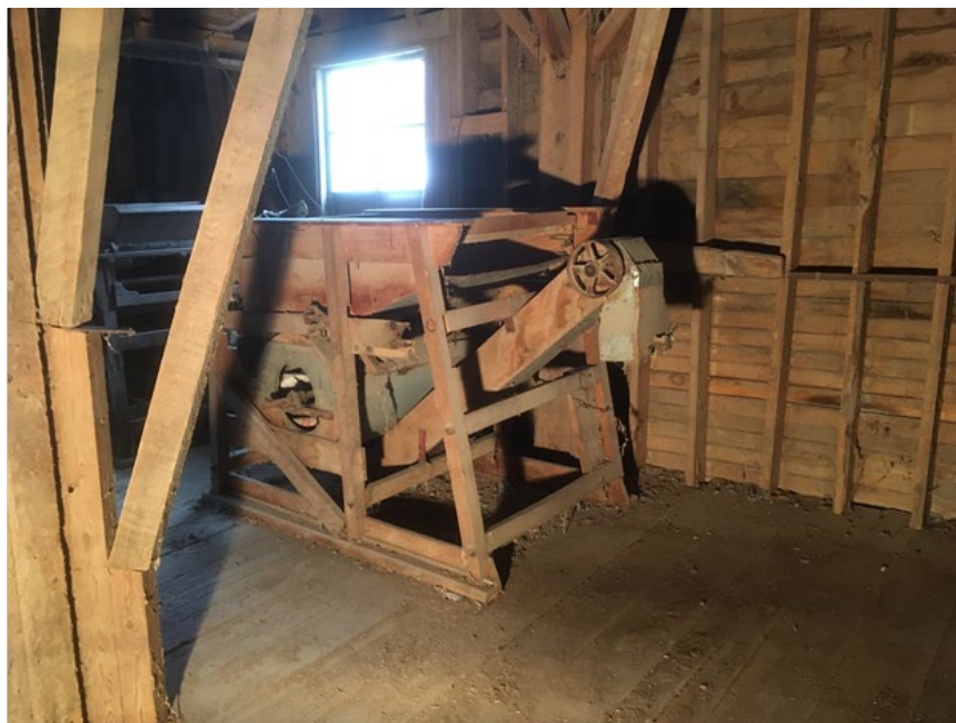
Photo #8 (MN_Fillmore County_Mc Michael Grain Elevator_0008) Interior view of fanning mill and working house framing.
