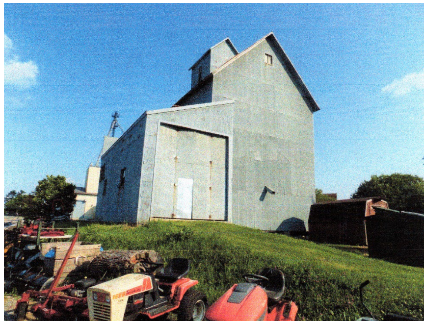
Photo #5 (MN_Fillmore County_Mc Michael Grain Elevator_0005) View of drive shed and west elevation. Facing east.
