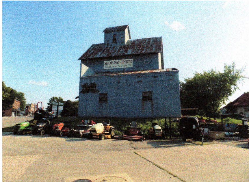
Photo #4 (MN_Fillmore County_Mc Michael Grain Elevator_0004) View of drive shed and north elevation, Main Avenue North visible on the left. Facing south
