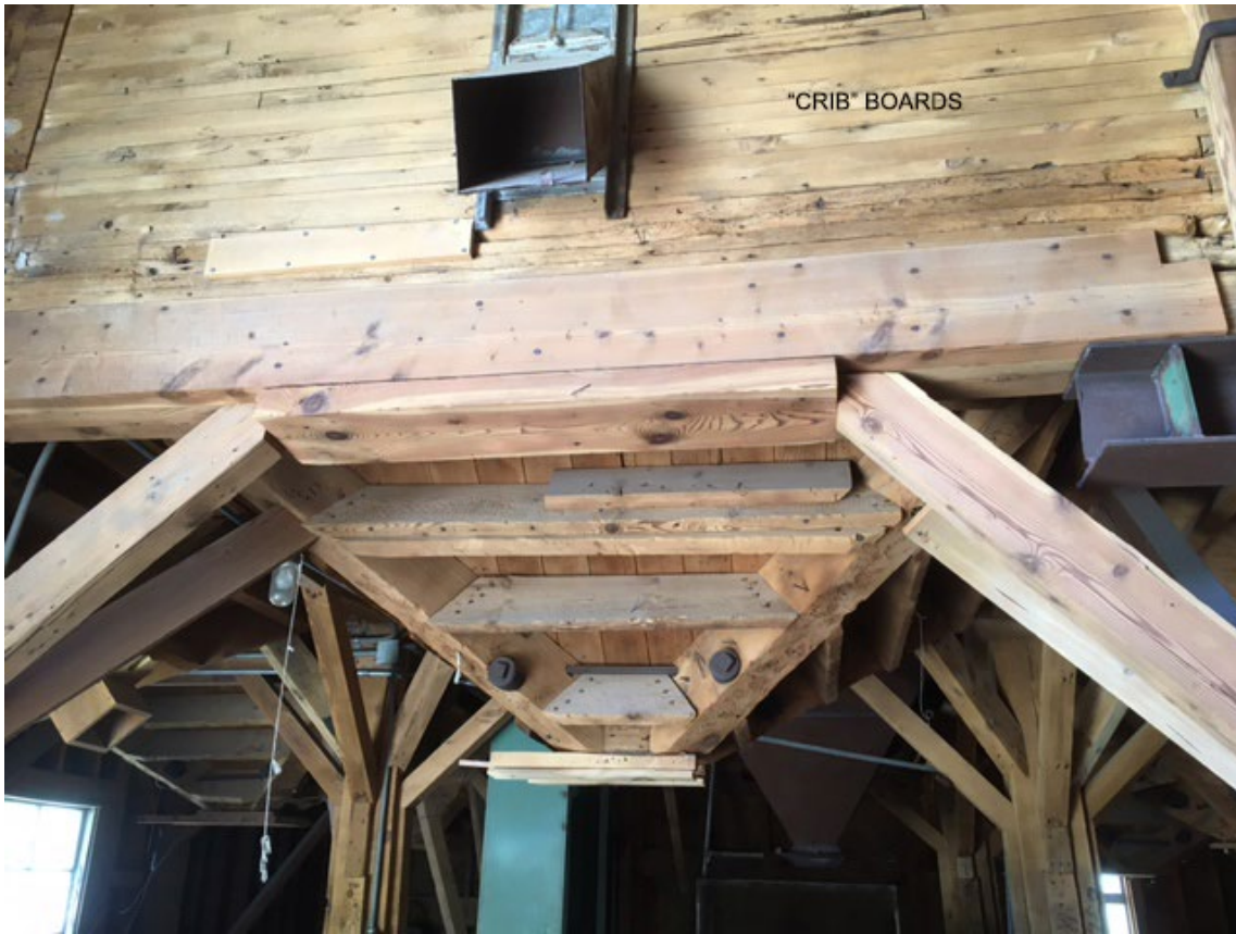
Photo #6 (MN_Fillmore County_Mc Michael Grain Elevator_0006) Interior view of the bottom of the grain bin showing "crib" board construction.
