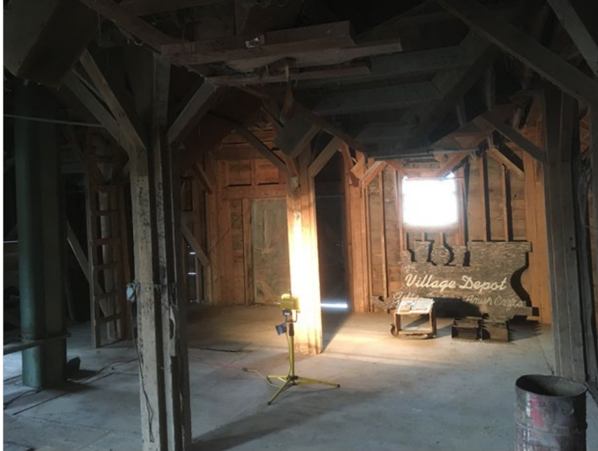
Photo #7 (MN_Fillmore County_Mc Michael Grain Elevator_0007) Interior view of working house framing.
