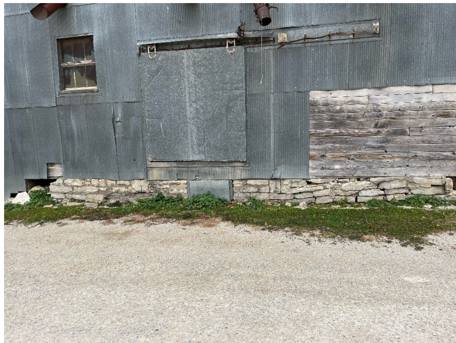
Photo #12 (MN_Fillmore County_Mc Michael Grain Elevator_00012) Fieldstone foundation.
