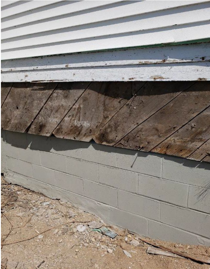
Figure 7: Immanuel Lutheran Church original timber cladding exposed for repairs during foundation rebuild in 2020. Photo Linda Leraas Ray, 2020.
