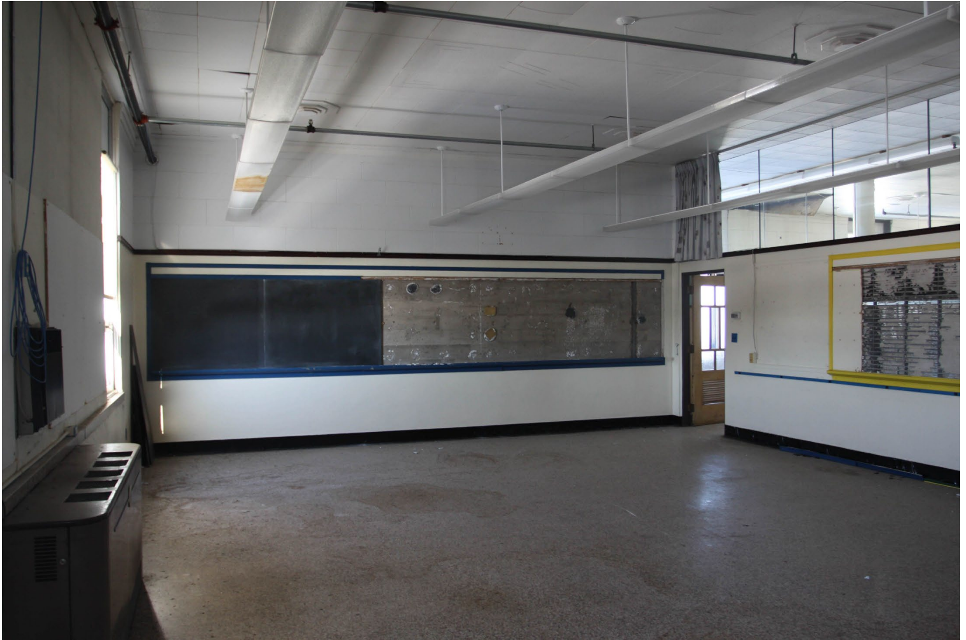
MN_Todd County_Eagle Bend High School_0013 Classroom building, second-floor classroom, looking northeast.
