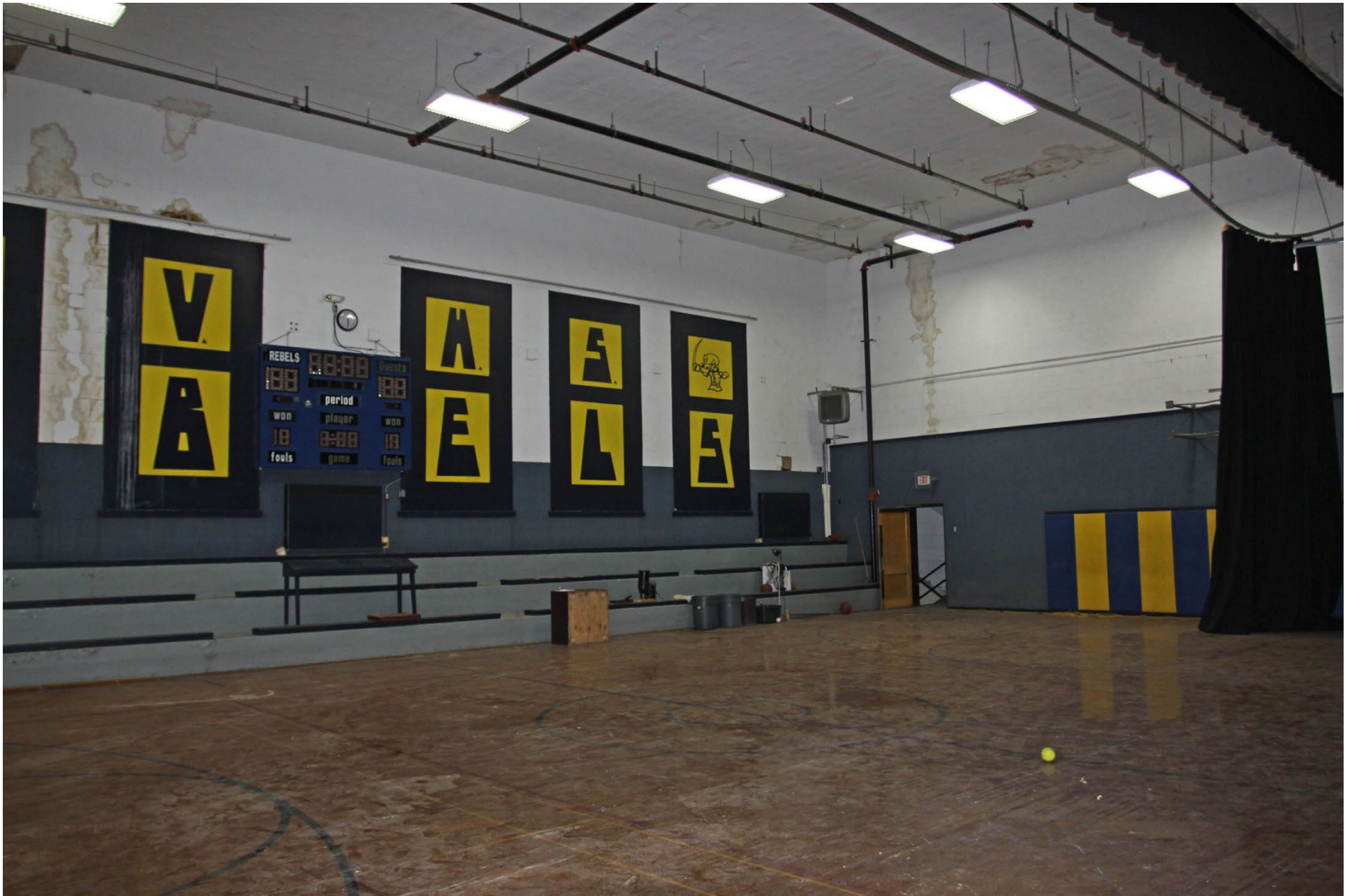
MN_Todd County_Eagle Bend High School_0009 Auditorium stage, looking northwest.
