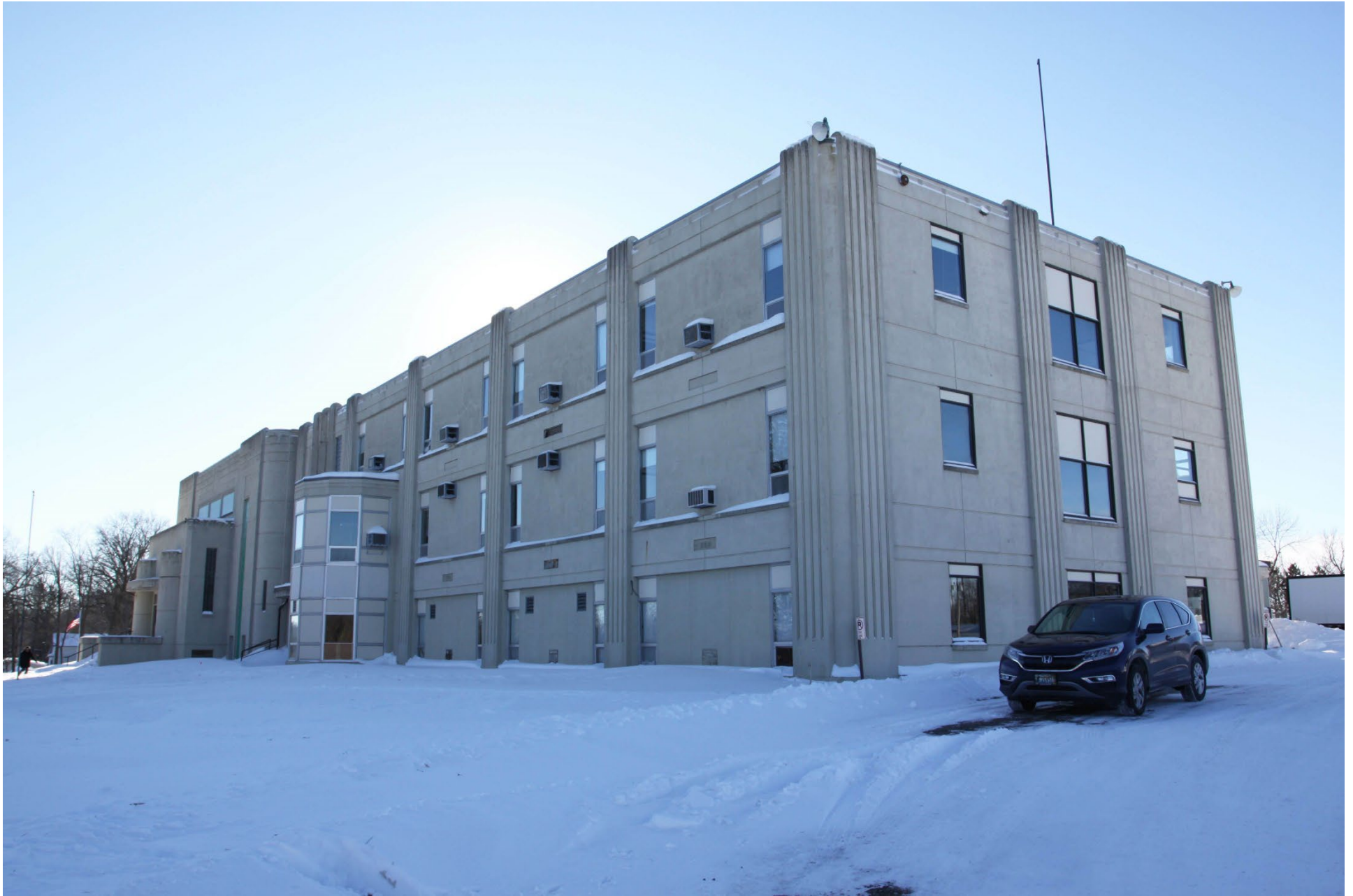
MN_Todd County_Eagle Bend High School_0004 East (left) and north (right) façades, looking southwest.
