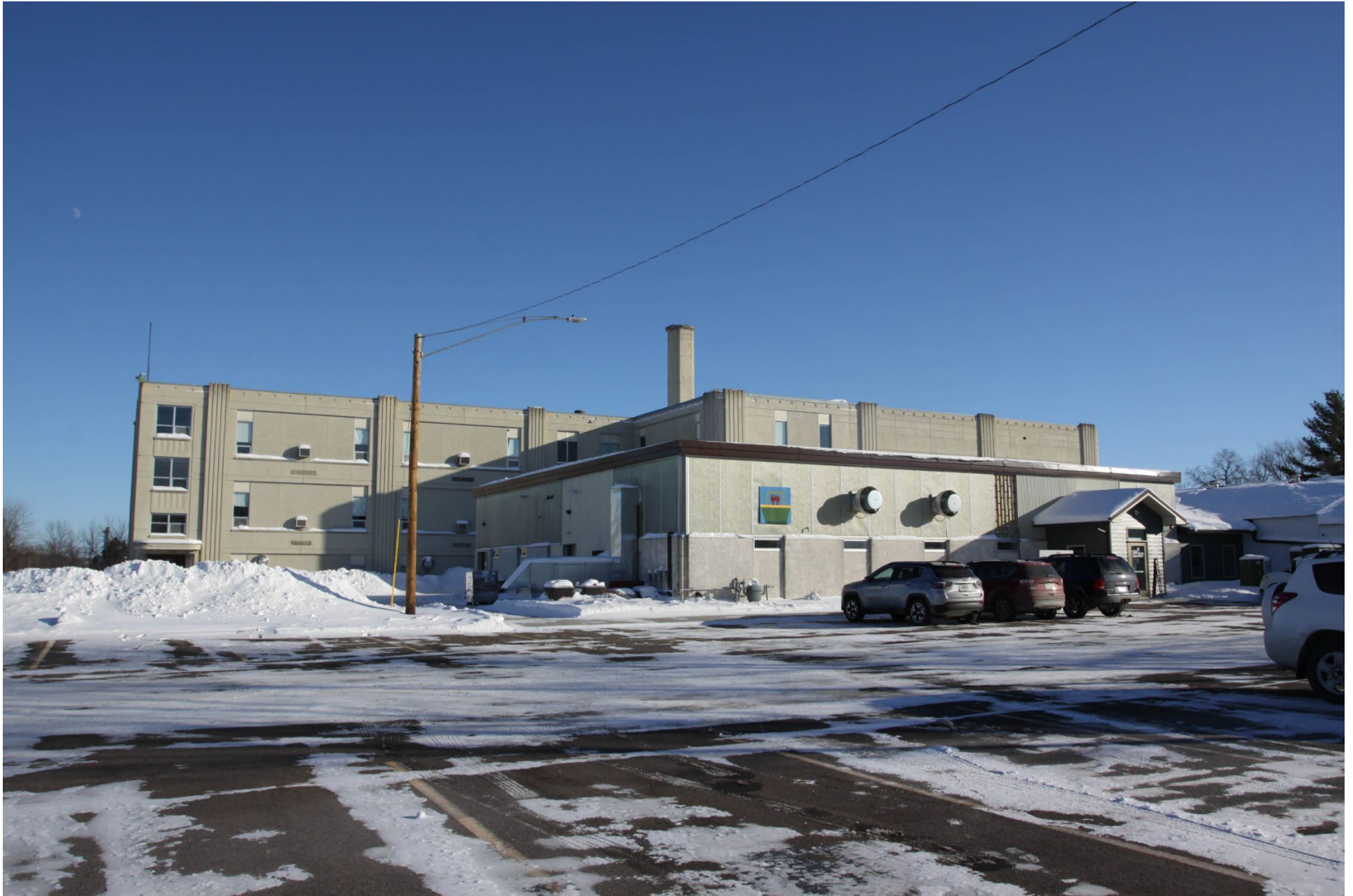
MN_Todd County_Eagle Bend High School_0005 West façade and non-historic 1964 addition, looking southeast.
