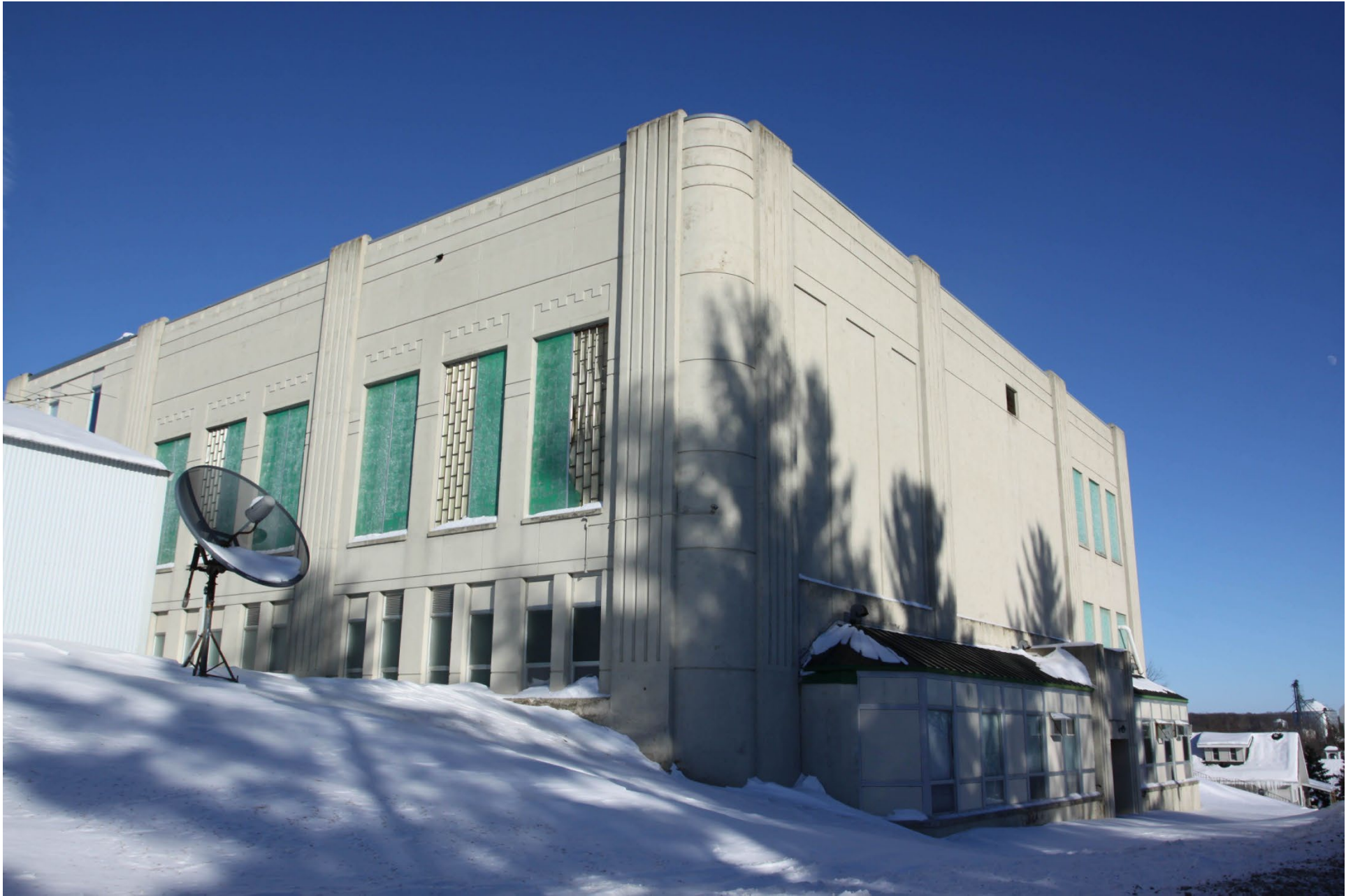
MN_Todd County_Eagle Bend High School_0007 West façade (left) and south façade (right), looking northeast.
