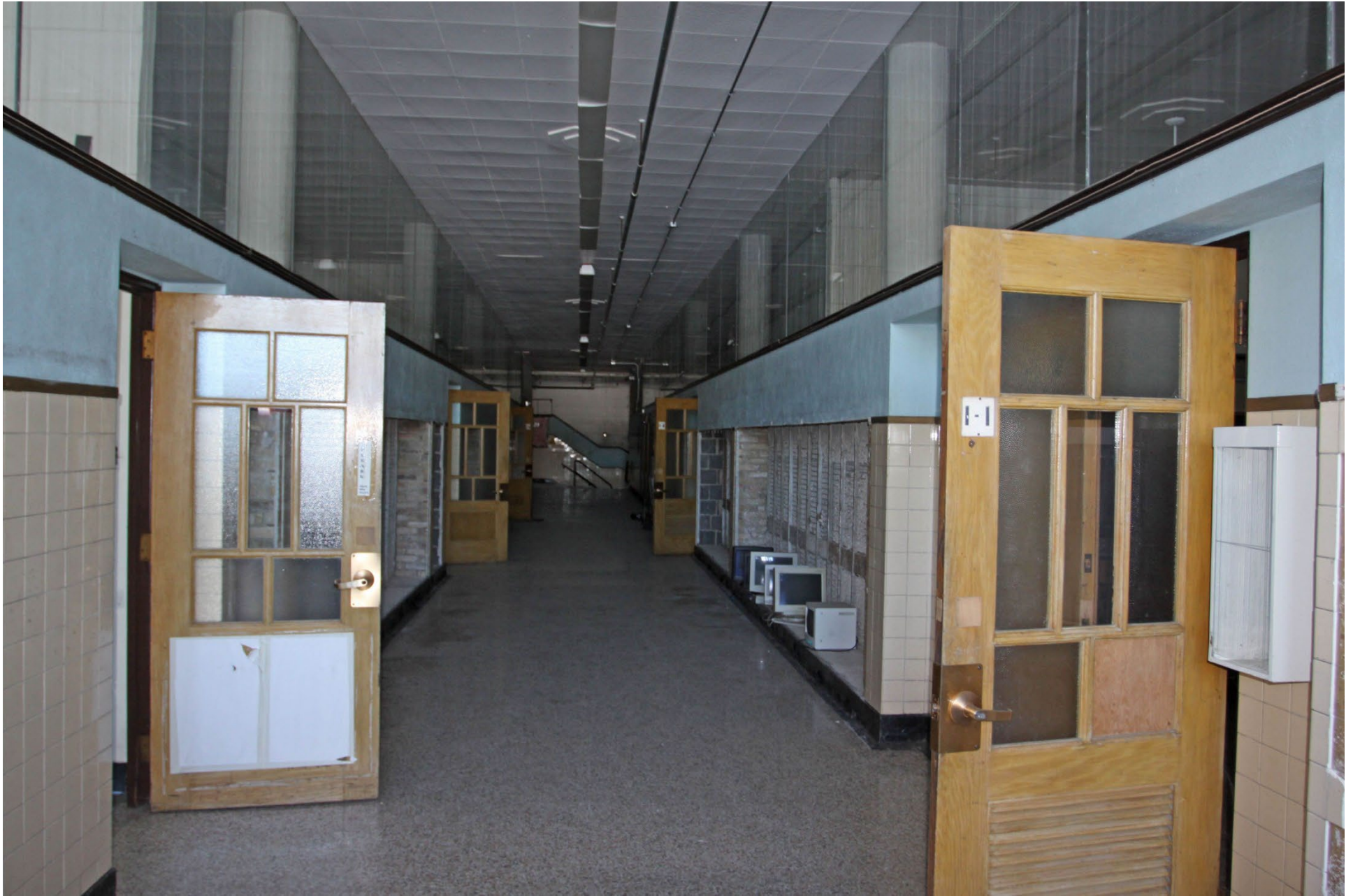
MN_Todd County_Eagle Bend High School_0011 Classroom building, ground-floor corridor, looking south.
