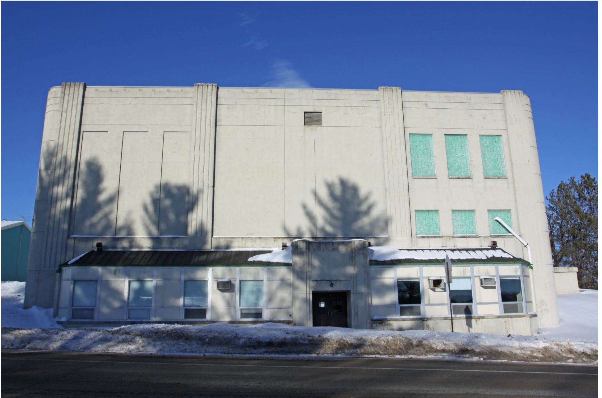
MN_Todd County_Eagle Bend High School_0006 South façade, looking north.
