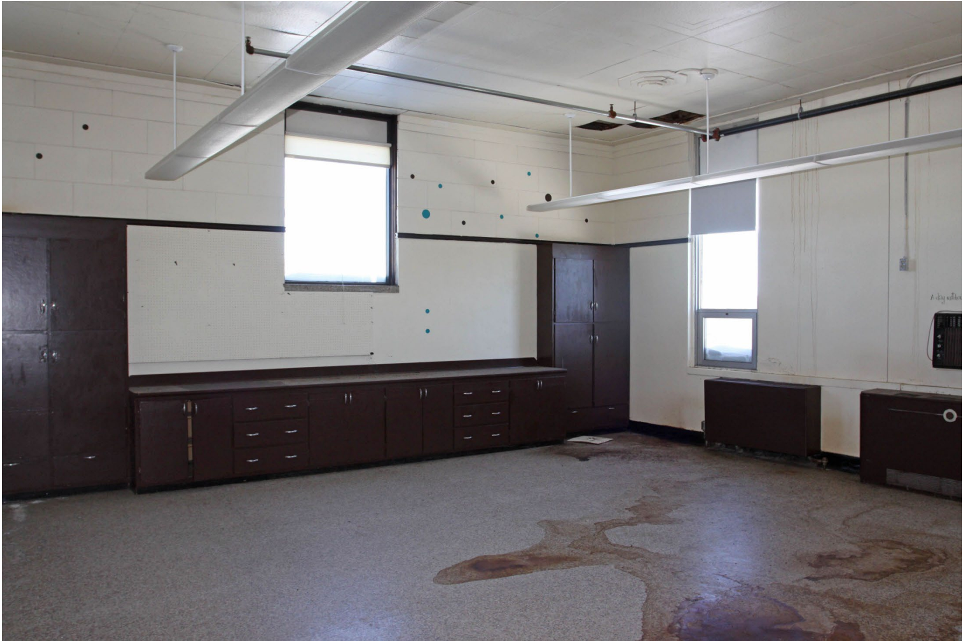
MN_Todd County_Eagle Bend High School_0014 Classroom building, second-floor classroom, looking northeast.
