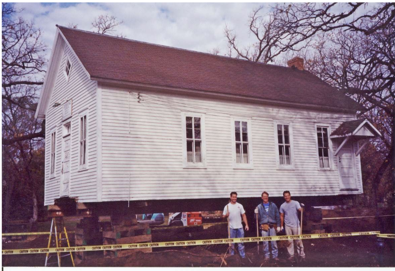
Figure G: Rebuilding the school foundation, 2003. Courtesy of the Champlin Historical Society.
