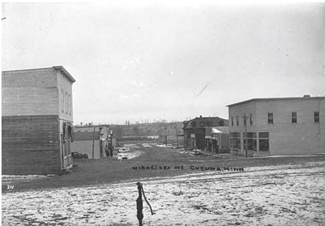
Images 9 and 10. Top: Minnesota Avenue, facing north, ca. 1910. The three-story Cuyuna Hotel with the Mansard roof is at center left. Bottom: Minnesota Avenue facing south, ca. 1910. Photos Minnesota Historical Society.
