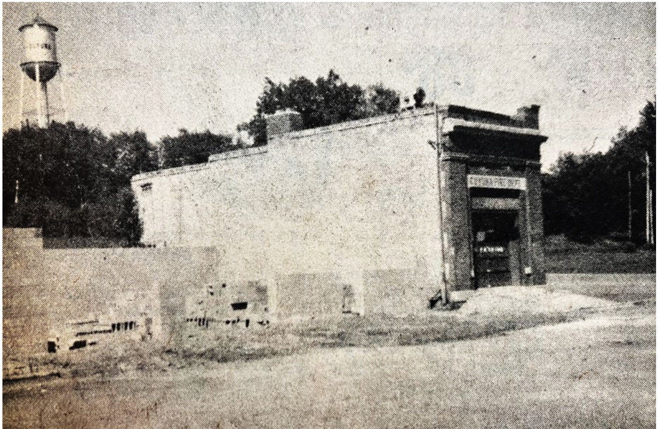
Image 16. Construction photograph of the 1978 addition, which is to the left of the 1911 building. Note the rising sections of concrete blocks that will flank the service and garage doors. Also note the rear wall, which is built into the hillside. Photo courtesy Crosby-Ironton Courier .
