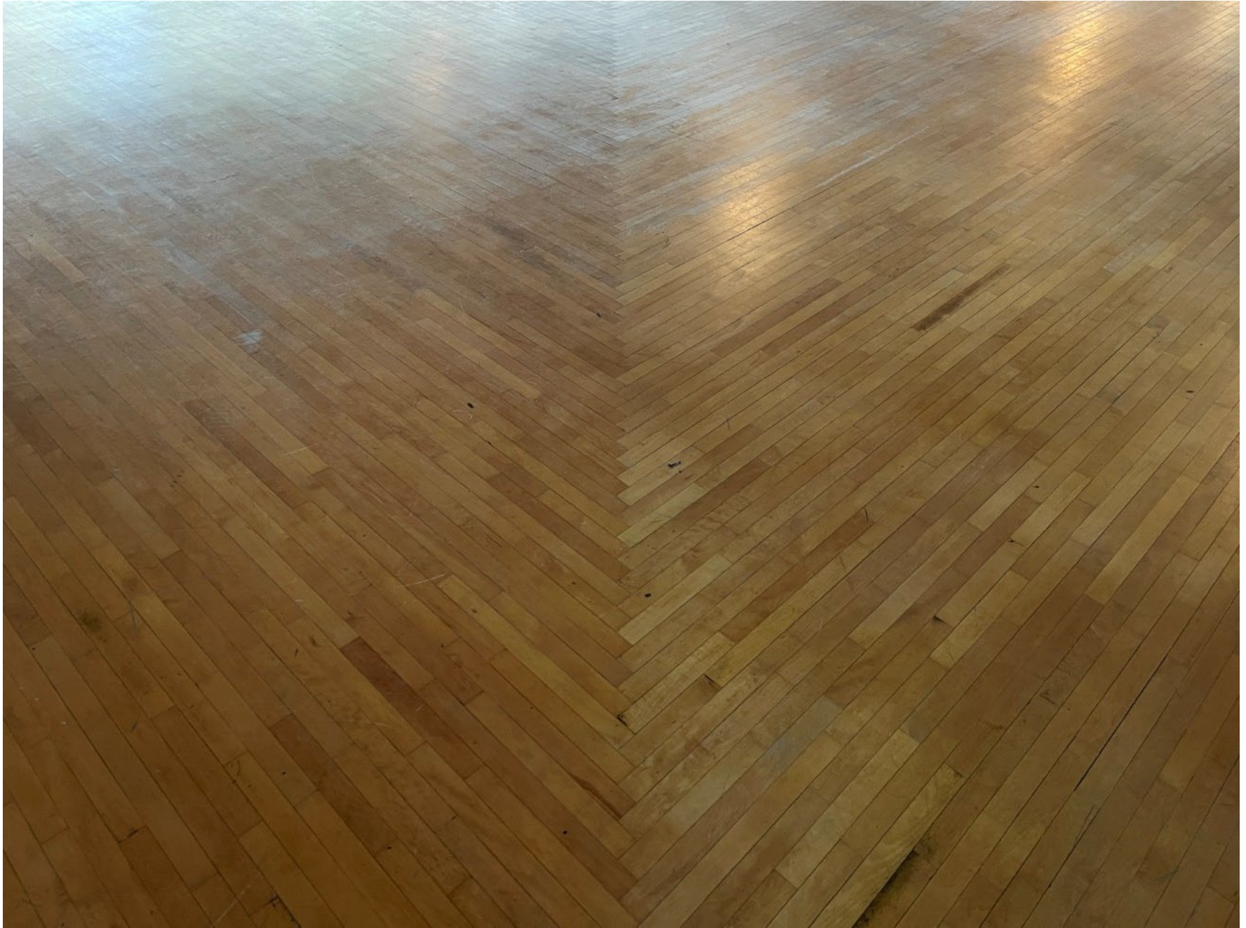
MN_Grant County_Barrett Lakeside Pavilion_0019 Interior view of the original dance floor, laid in a log-cabin pattern
