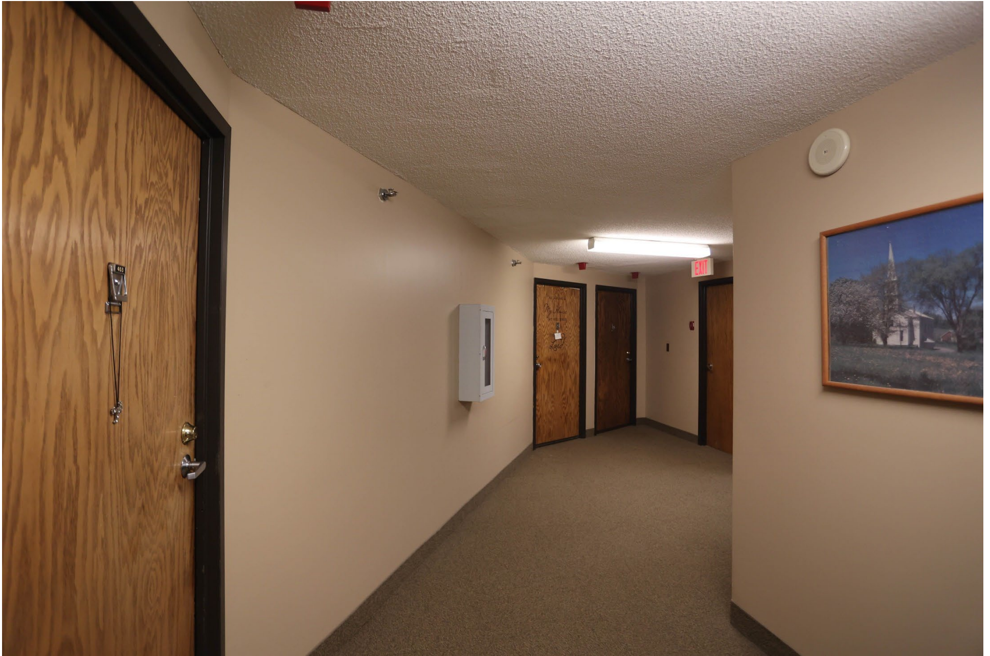
MN_Saint Louis County_Alice Nettell Tower_0008 fourth floor, hallway, looking east
