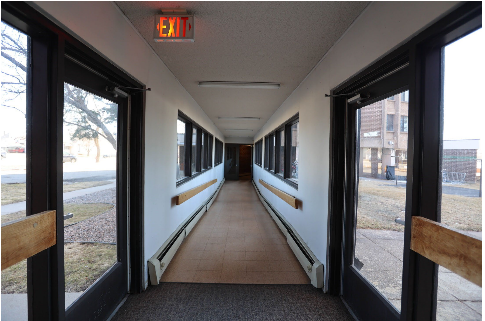
MN_Saint Louis County_Alice Nettell Tower_0004 first floor, breezeway, looking north
