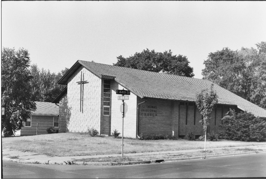
Figure 21. St. Thomas Episcopal Church, 1980 (4400 4th Avenue South, extant) 658
