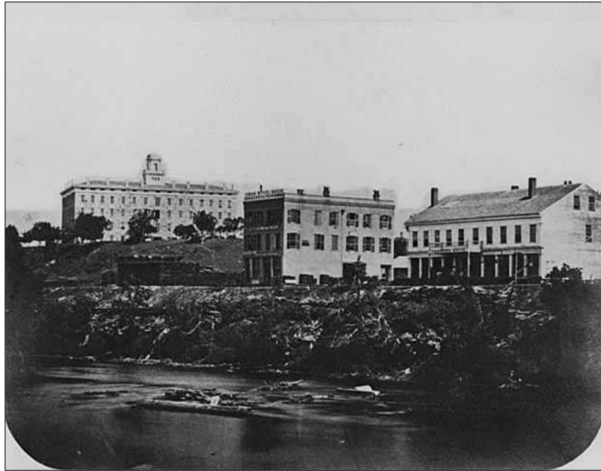
Figure 3. Winslow House (left, non-extant) and Jarrett House (right, non-extant) in 1858 640
