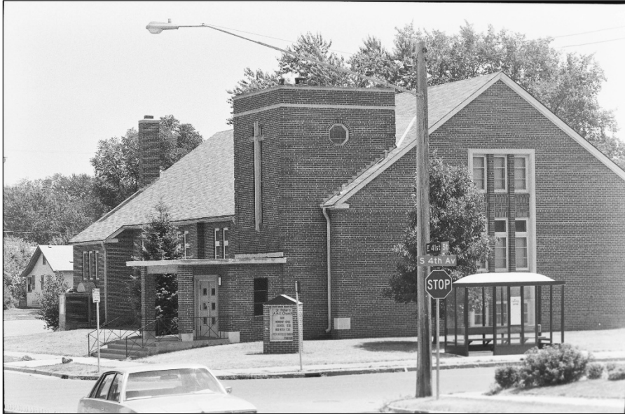
Figure 15. St. Peter's AME Church, 1980 (401 41st Street East, extant) 652
