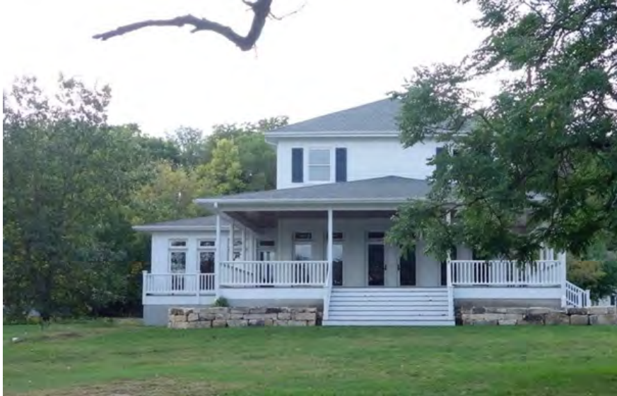
Figure 18. Lake-Side Hotel, later Frontenac Inn and Methodist Campus Dining Hall. Photograph 2021 after removal of upper story and conversion to a single-family dwelling. (C. Zellie 2021)
