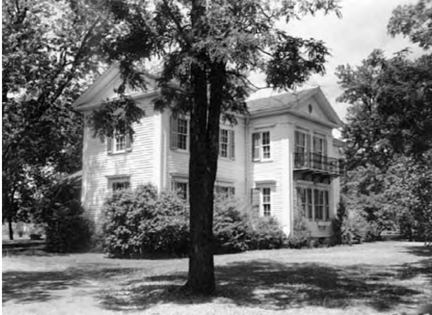
Figure 9. Locust Lodge (1861; GD-FLC-025), in 1959. (MHS)
