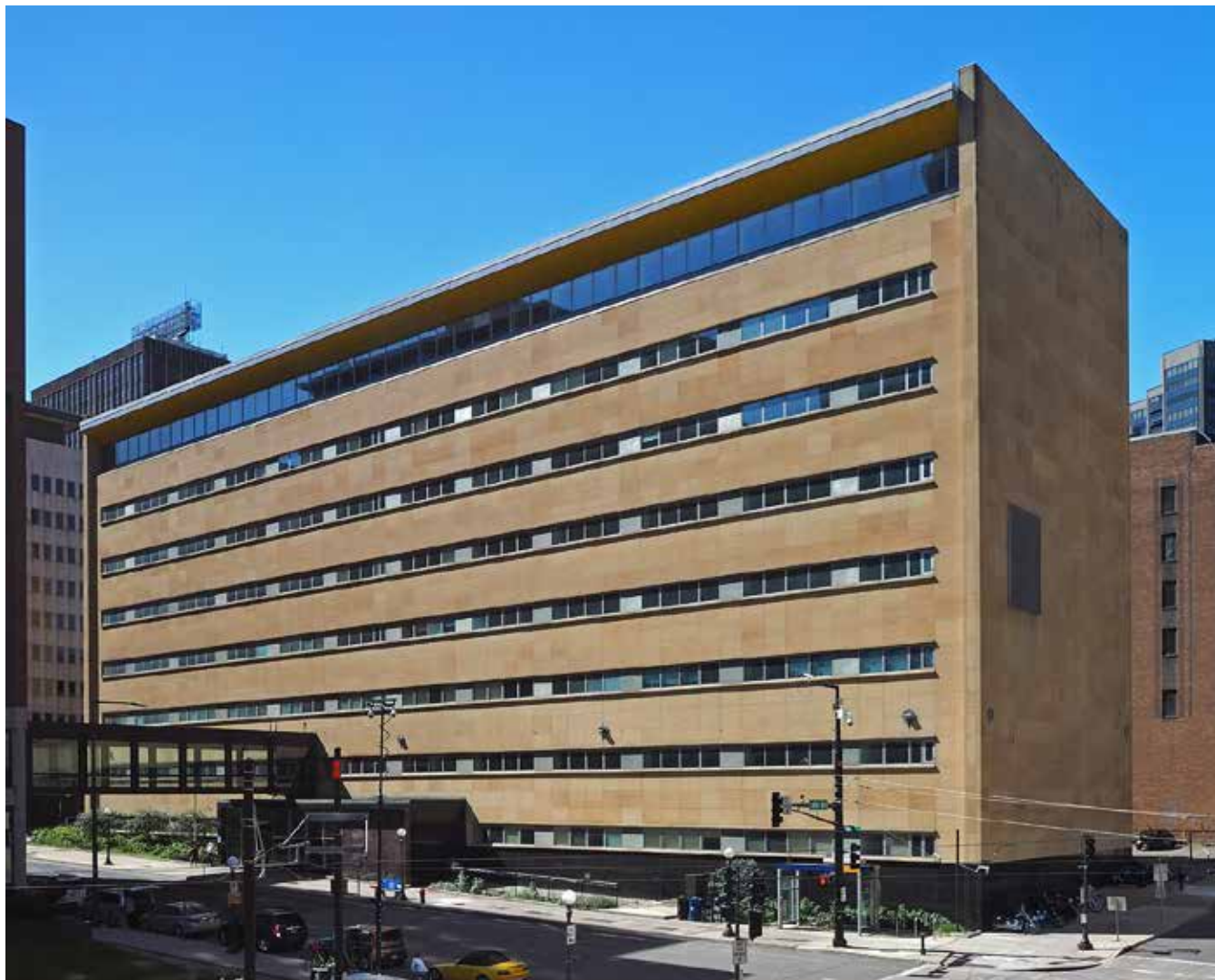
Figure 5. Minnesota Mutual Life Insurance Company, Ellerbee and Company, 1955. Photograph courtesy of Wikimedia Commons.
