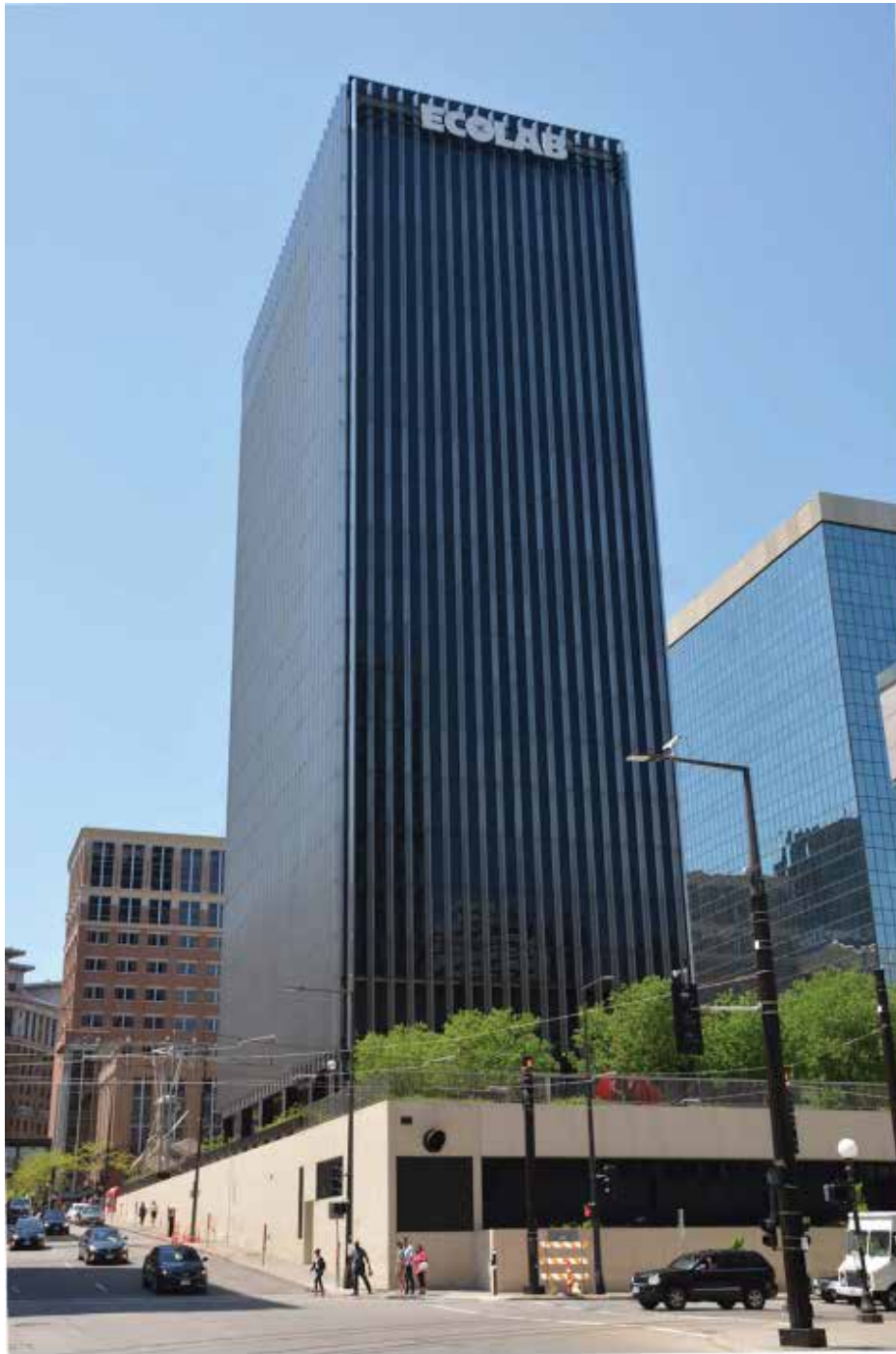
Figure 7. Osborn Building, Bergstedt, Wahlberg and Wold, 1968. (Northern Federal Building in background right of image). Photograph by Amy Lucas, Osborn Building NRHP Nomination, #100003233.
