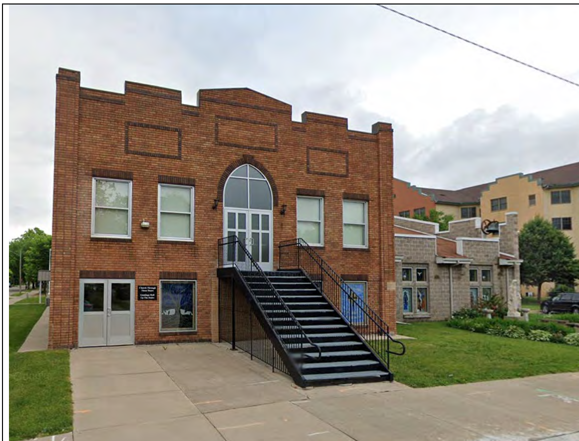
Figure N Church of St. Hedwig, 129 29 th Street Northeast, 2019. Google Maps.
