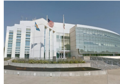
Public Safety Building New Castle County, DE
