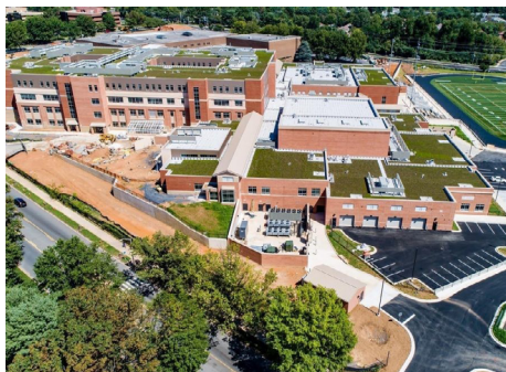
Seneca Valley High School Commissioning Germantown, MD
