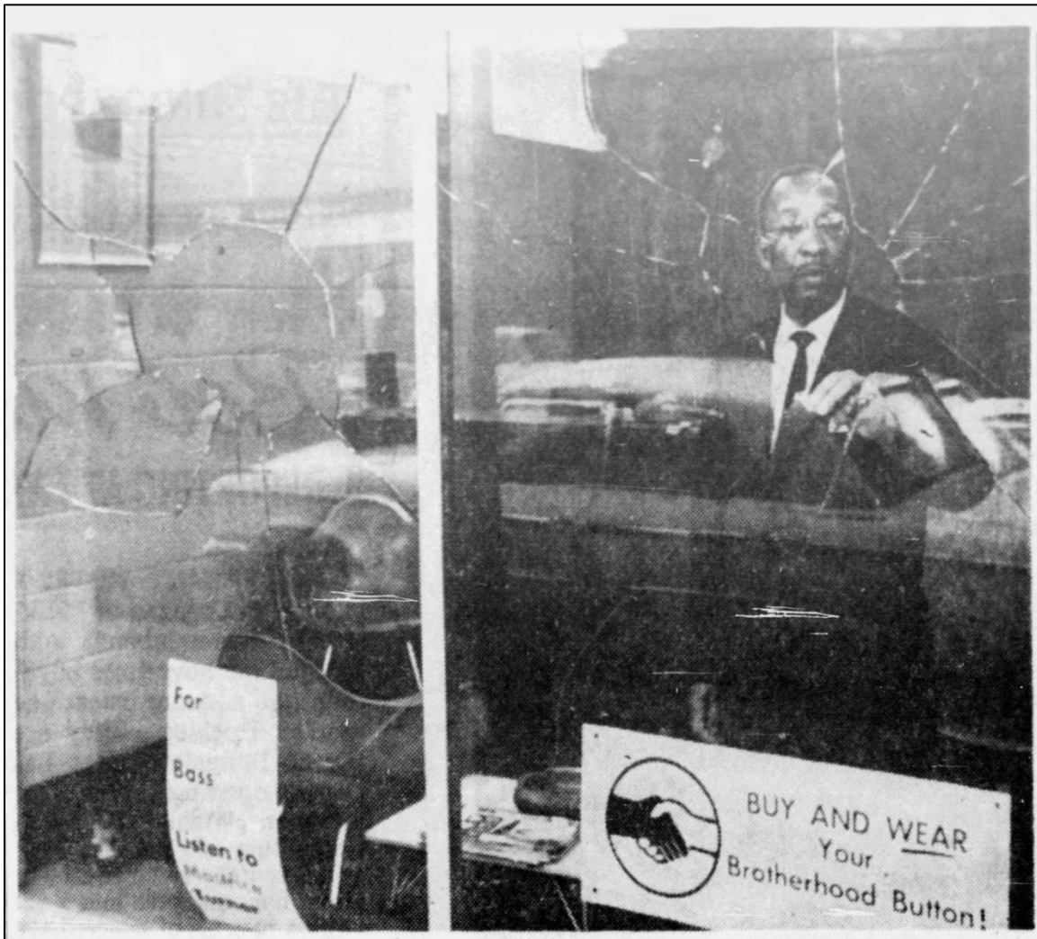
Figure 11. Newman inspecting damage to the building's primary facade near the main entrance, which was the result of vandalism, in 1964. ( Minneapolis Star , August 31, 1964)
