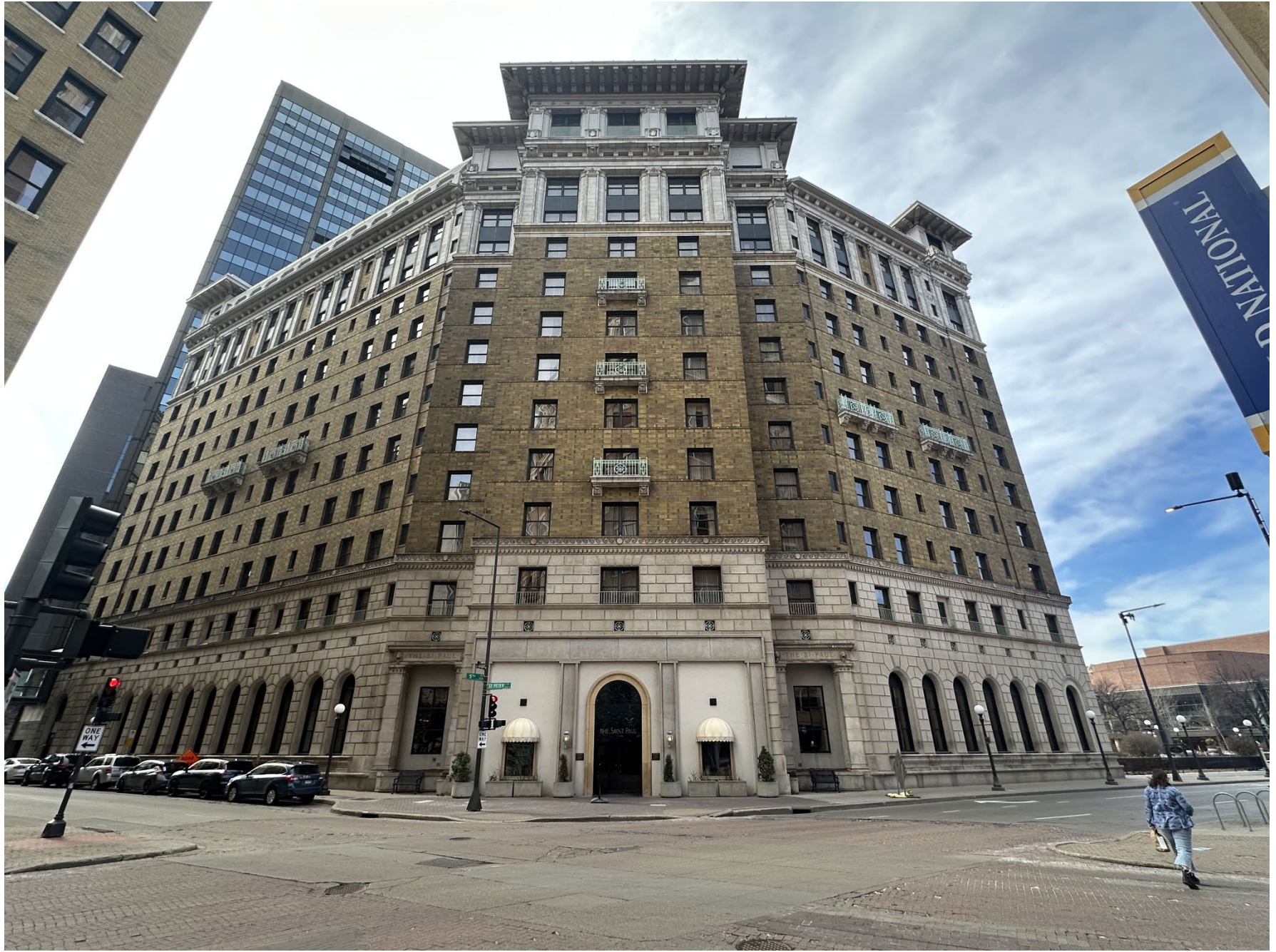
MN_Ramsey County_Saint Paul Hotel_0005 East and northeast elevations, camera facing south.
