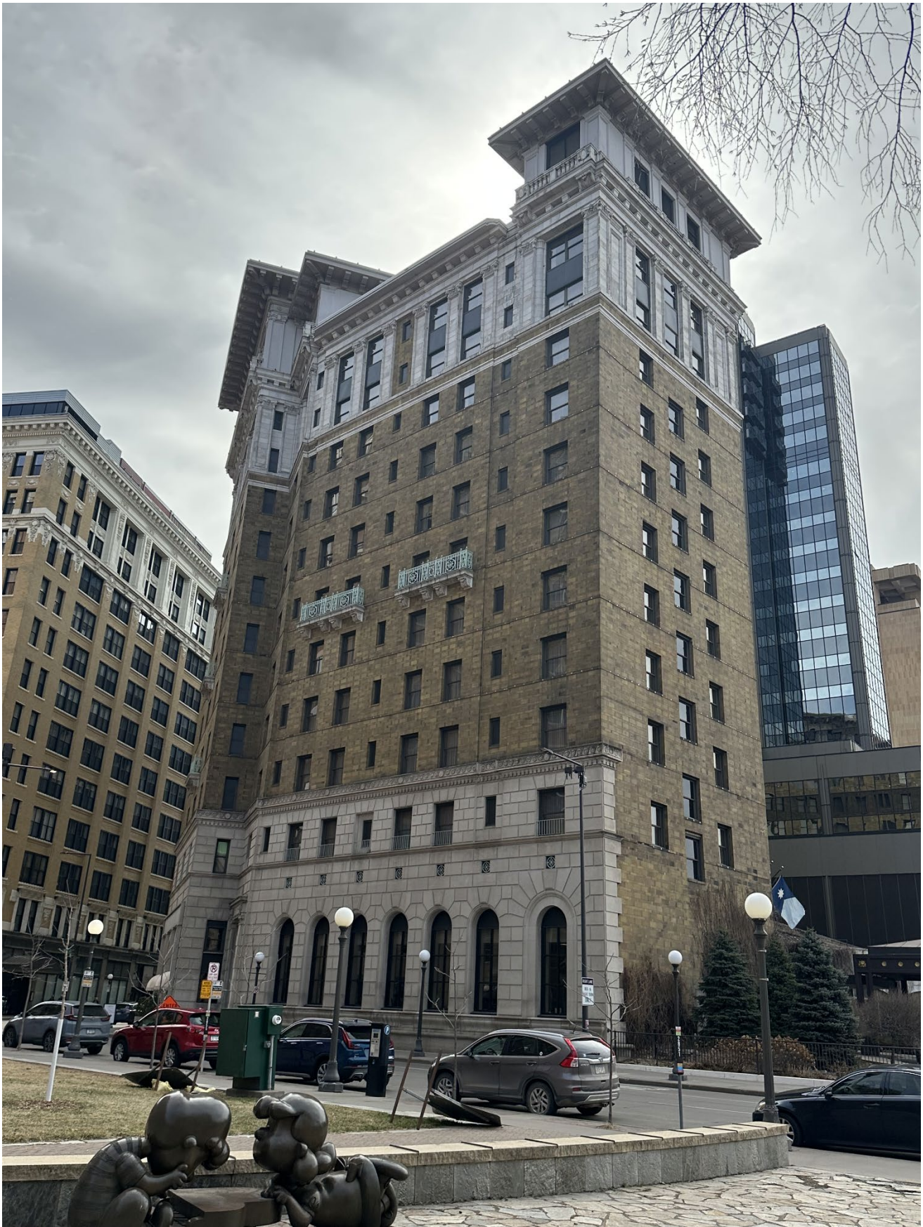
MN_Ramsey County_Saint Paul Hotel_0003 North and west elevations, camera facing southeast.
