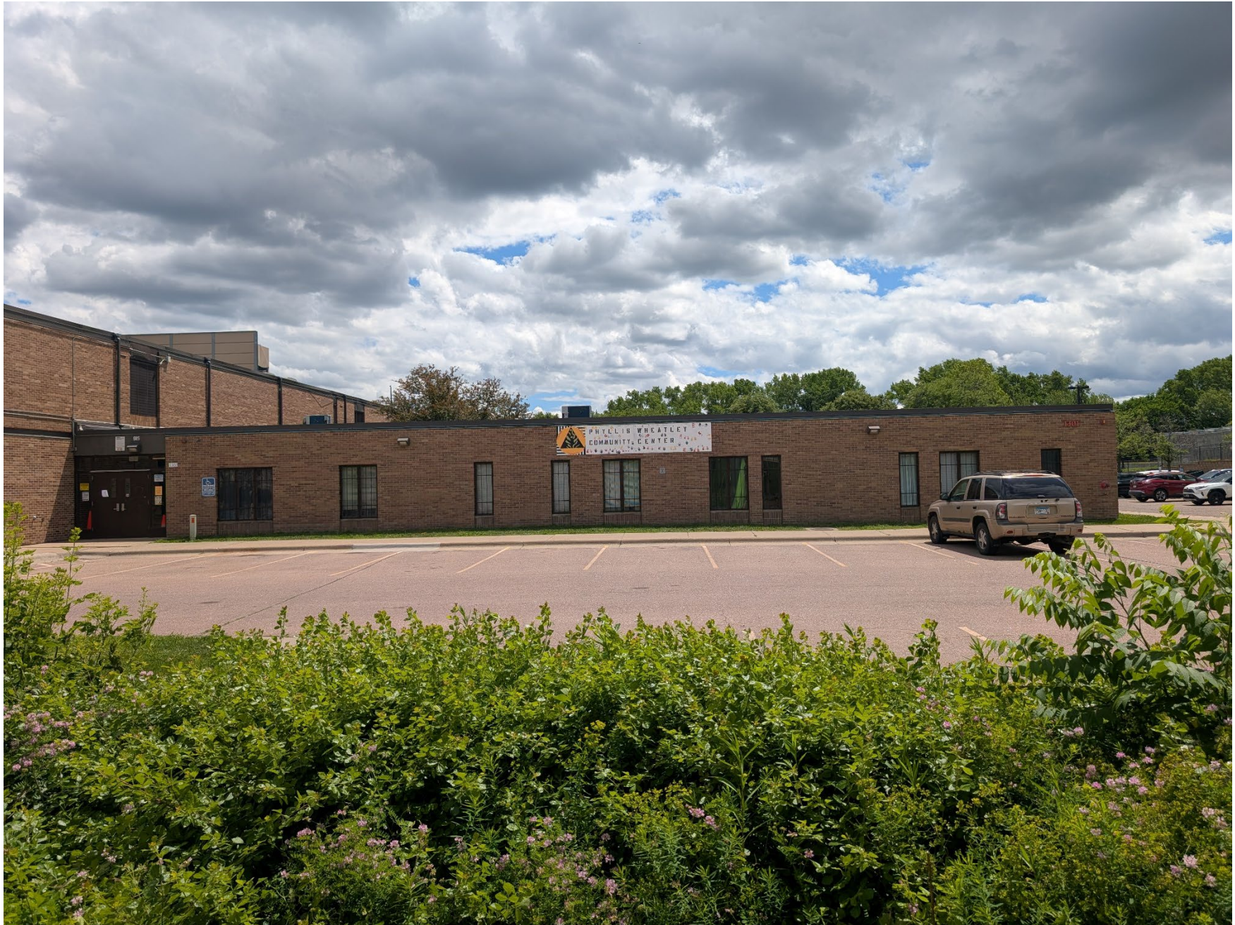
MN_Hennepin County_Phyllis Wheatley Community Center_0004 View of north elevation of Phyllis Wheatley Community Center, looking south.
