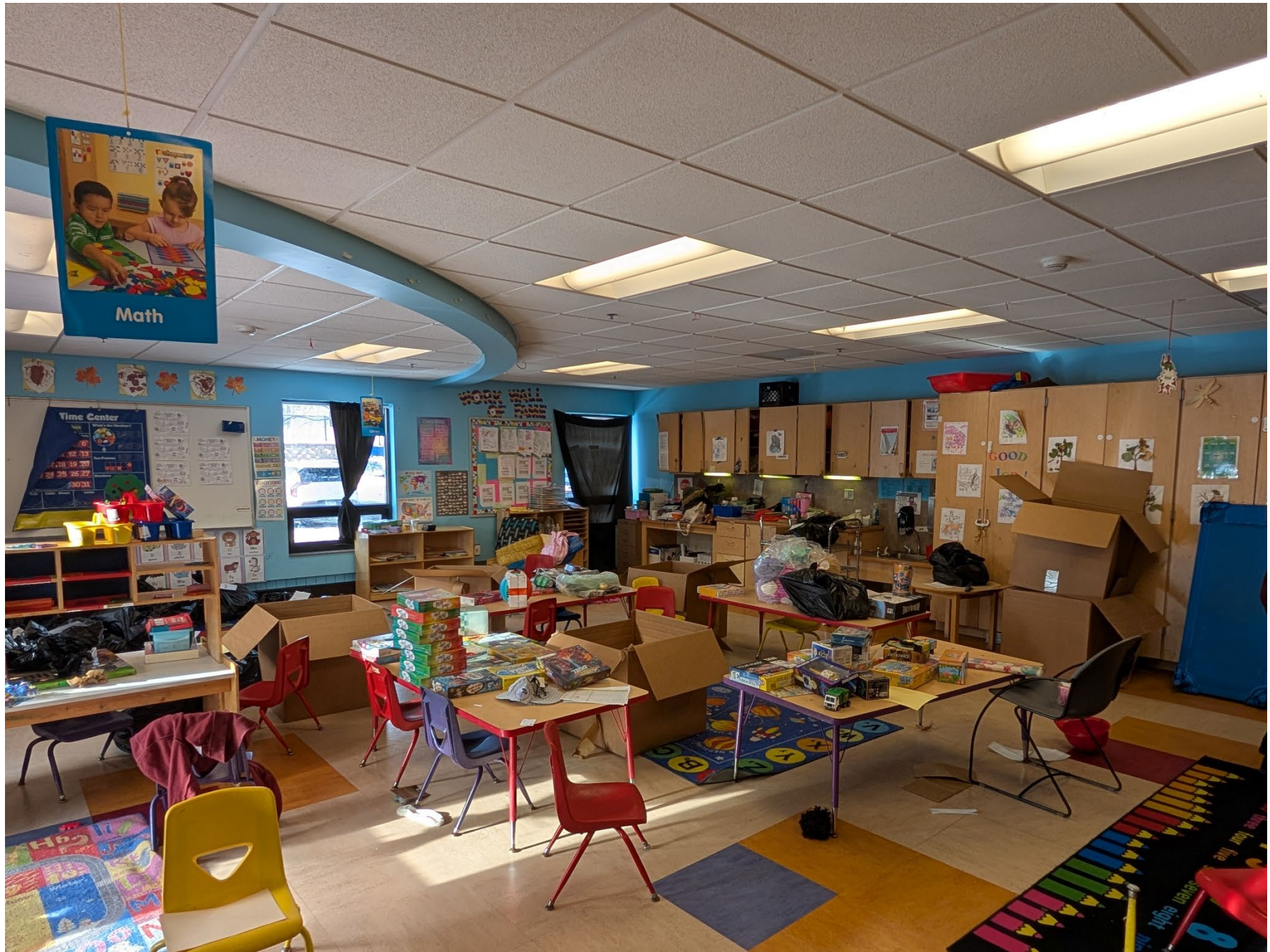
MN_Hennepin County_Phyllis Wheatley Community Center_0012 View of a classroom on the first level of Phyllis Wheatley Community Center, looking northwest.
