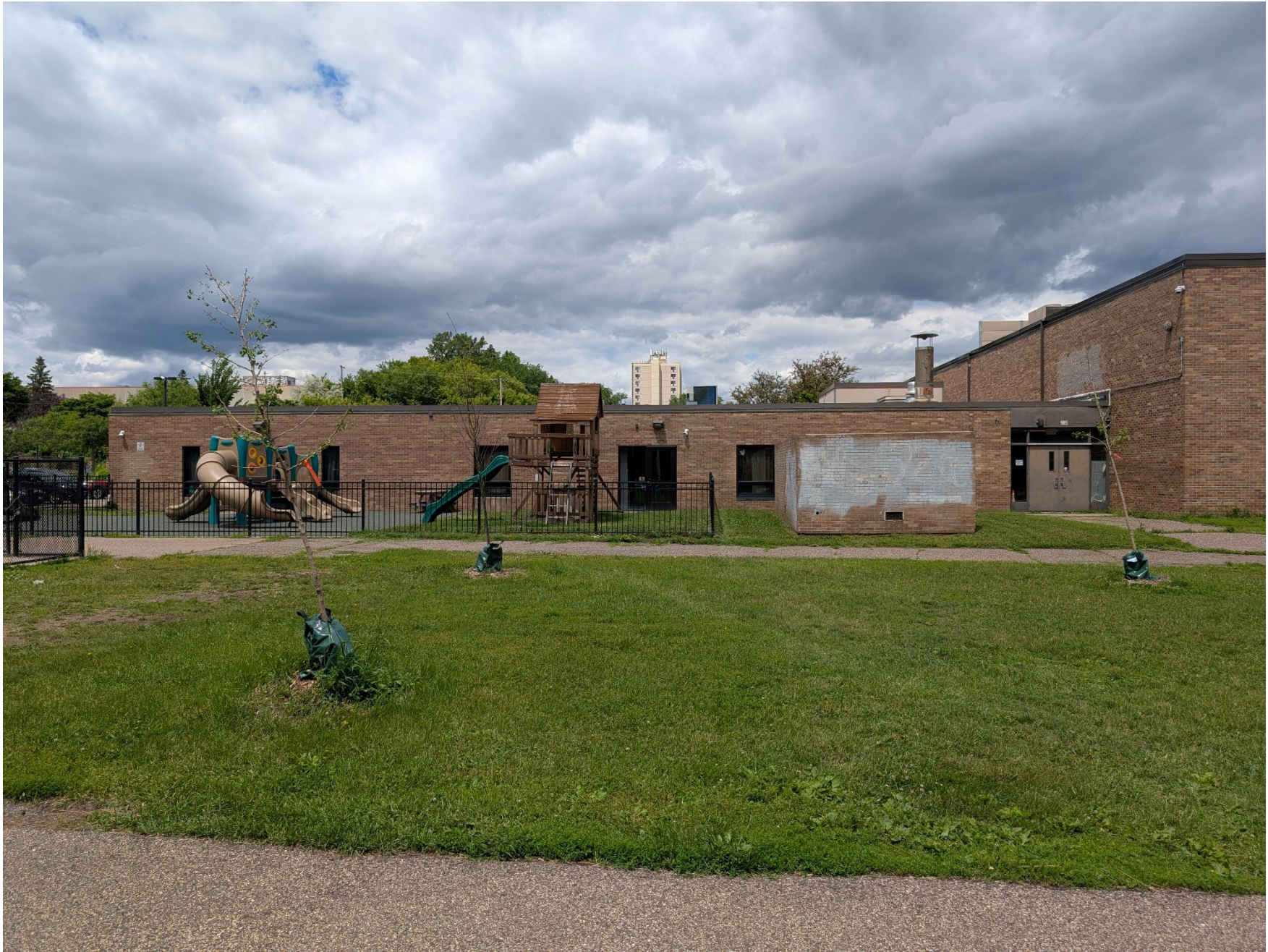
MN_Hennepin County_Phyllis Wheatley Community Center_0003 View of south elevation of Phyllis Wheatley Community Center, looking north.
