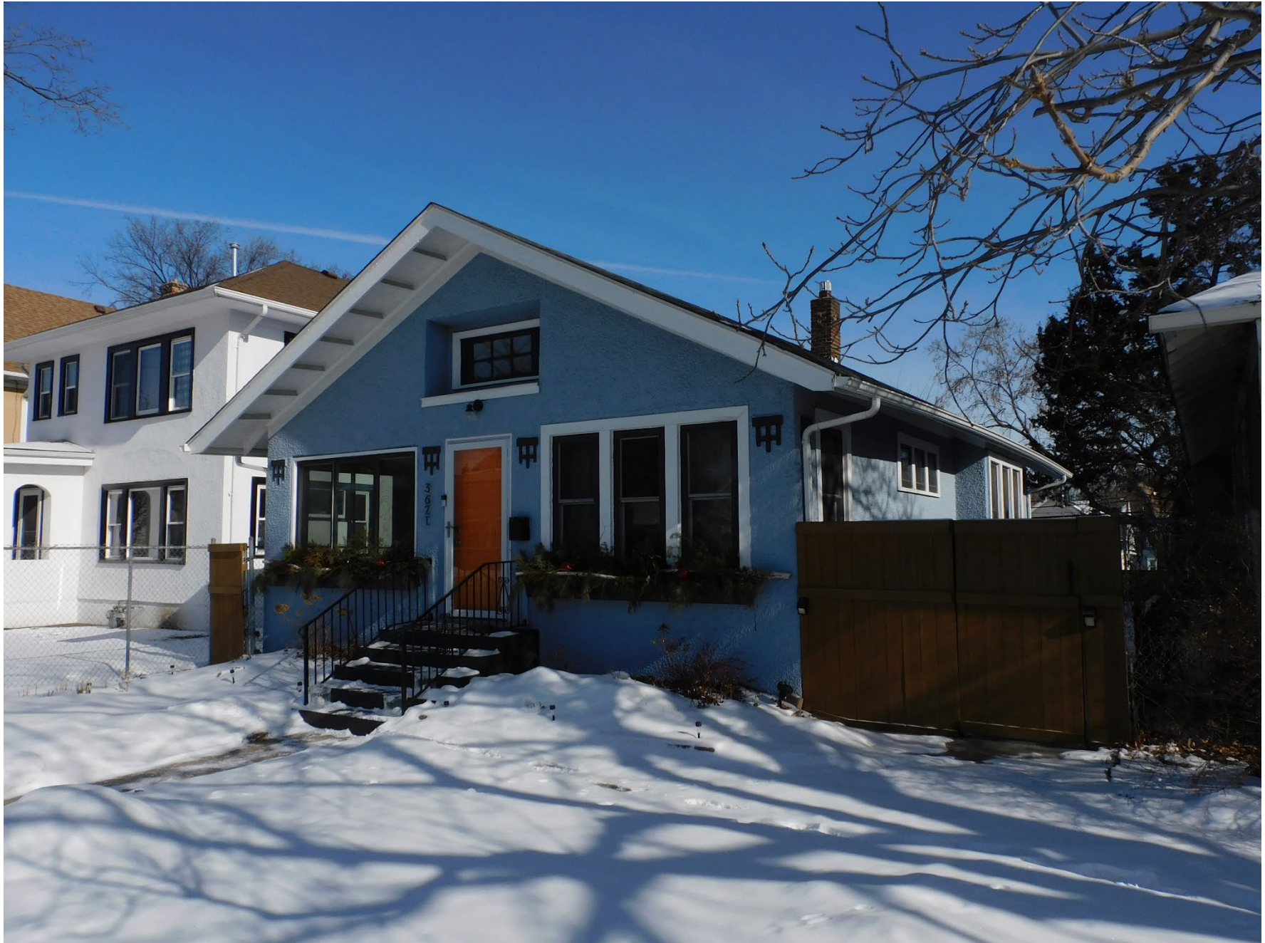
MN_Hennepin County_Davis, Harry, Sr. and Charlotte, House_0001 Overview of the Harry Davis, Sr. and Charlotte Davis House, view facing northeast.
