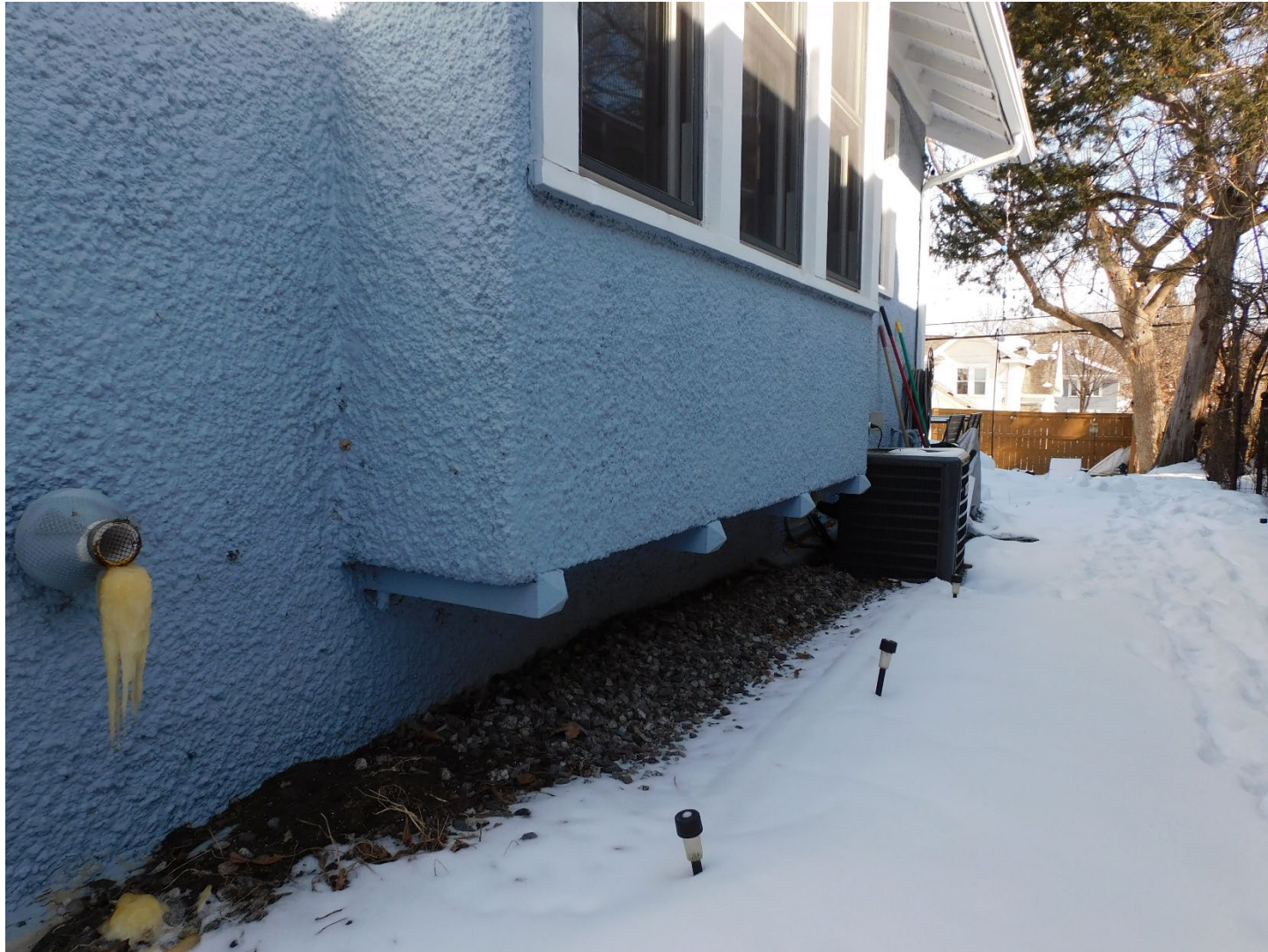
MN_Hennepin County_Davis, Harry, Sr. and Charlotte, House_0008 Oriel detail on south elevation, view facing northeast.
