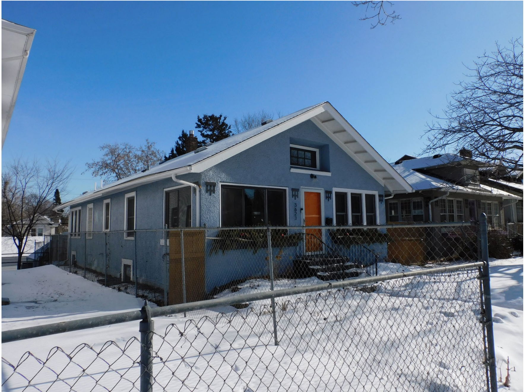
MN_Hennepin County_Davis, Harry, Sr. and Charlotte, House_0003 West (primary) façade and north elevation, view facing southeast.
