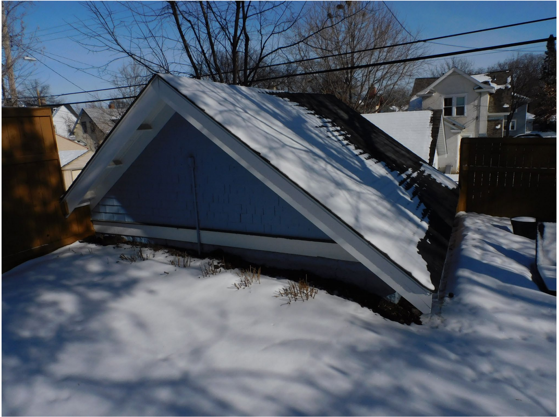
MN_Hennepin County_Davis, Harry, Sr. and Charlotte, House_0017 West elevation of garage, view facing east-northeast.
