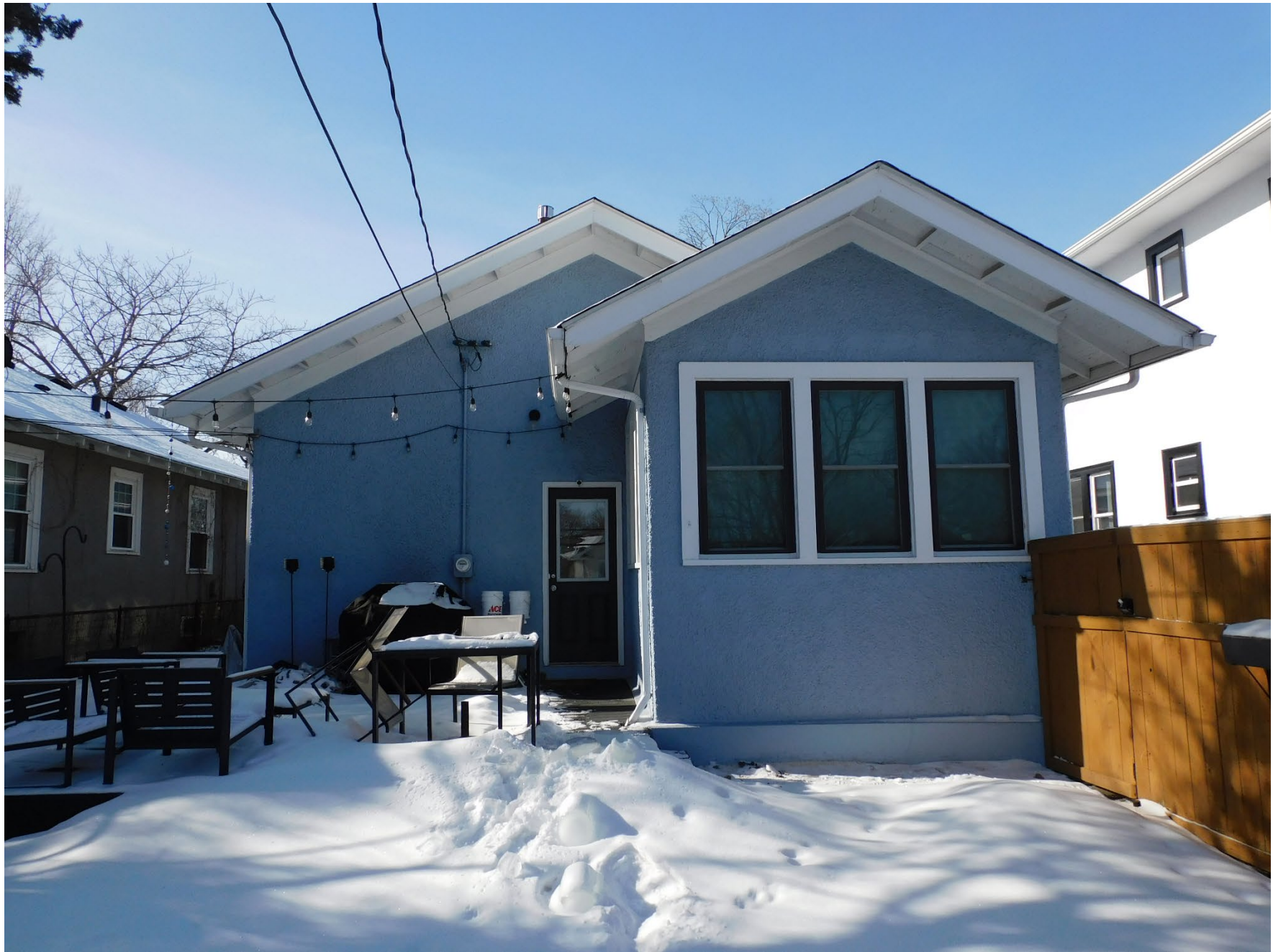
MN_Hennepin County_Davis, Harry, Sr. and Charlotte, House_0005 East elevation, view facing west.
