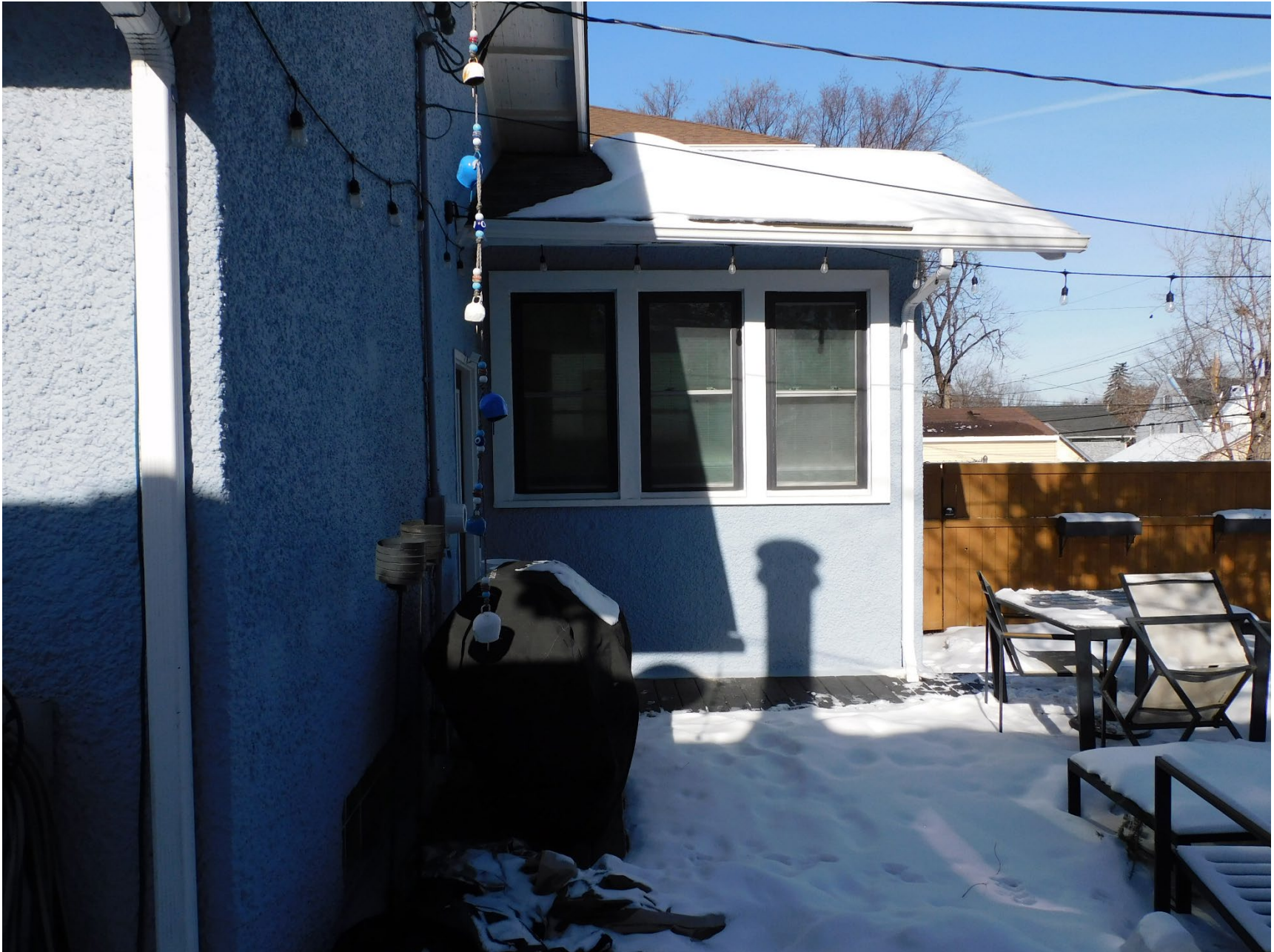
MN_Hennepin County_Davis, Harry, Sr. and Charlotte, House_0006 South elevation of wing on east elevation, view facing north.
