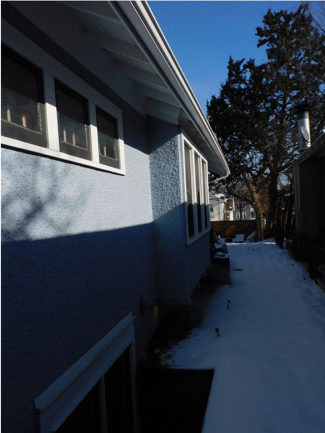
MN_Hennepin County_Davis, Harry, Sr. and Charlotte, House_0007 South elevation, view facing east-northeast.
