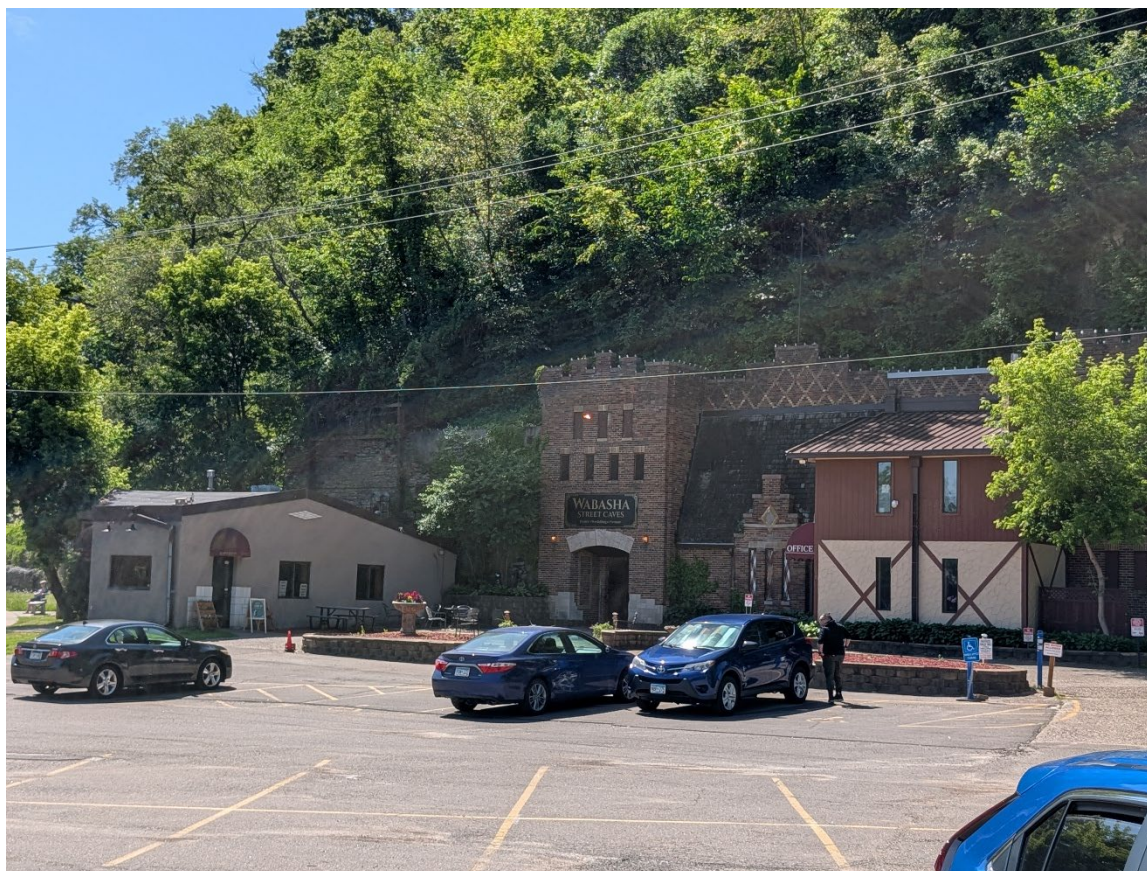
Figure AA. View of Wabasha Street Caves at 215 Wabasha Street South, looking south, June 2026.
