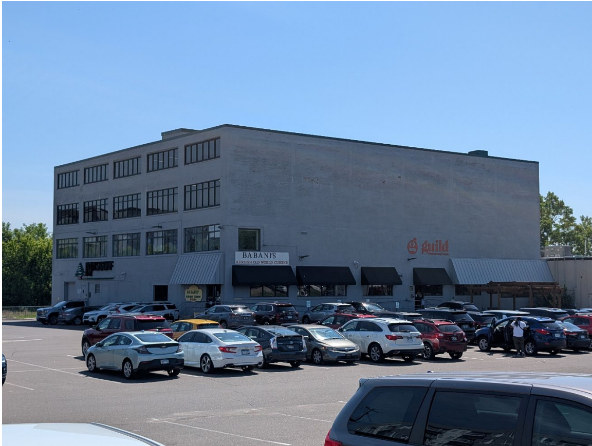
Figure FF. View of west and south elevations of the remaining building of the Cherry-Burrell Corporation, 34 Fillmore Avenue, looking northwest, June 2026.
