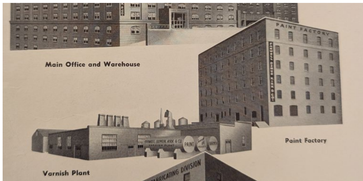
Figure U. View of the west and partial south elevation of Warehouse 2 (labeled "Paint Factory") and the varnish plant, from an FOK catalog, circa 1963. Image courtesy of Minnesota Historical Society.
