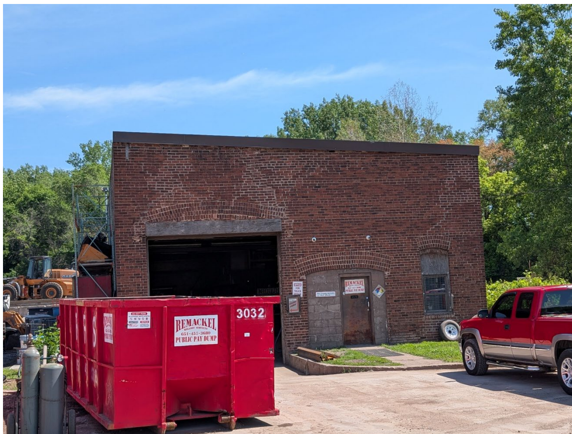
Figure HH. View of south elevation of the remaining building of the otherwise non-extant complex at 565 Barge Channel Road, looking north, June 2026.
