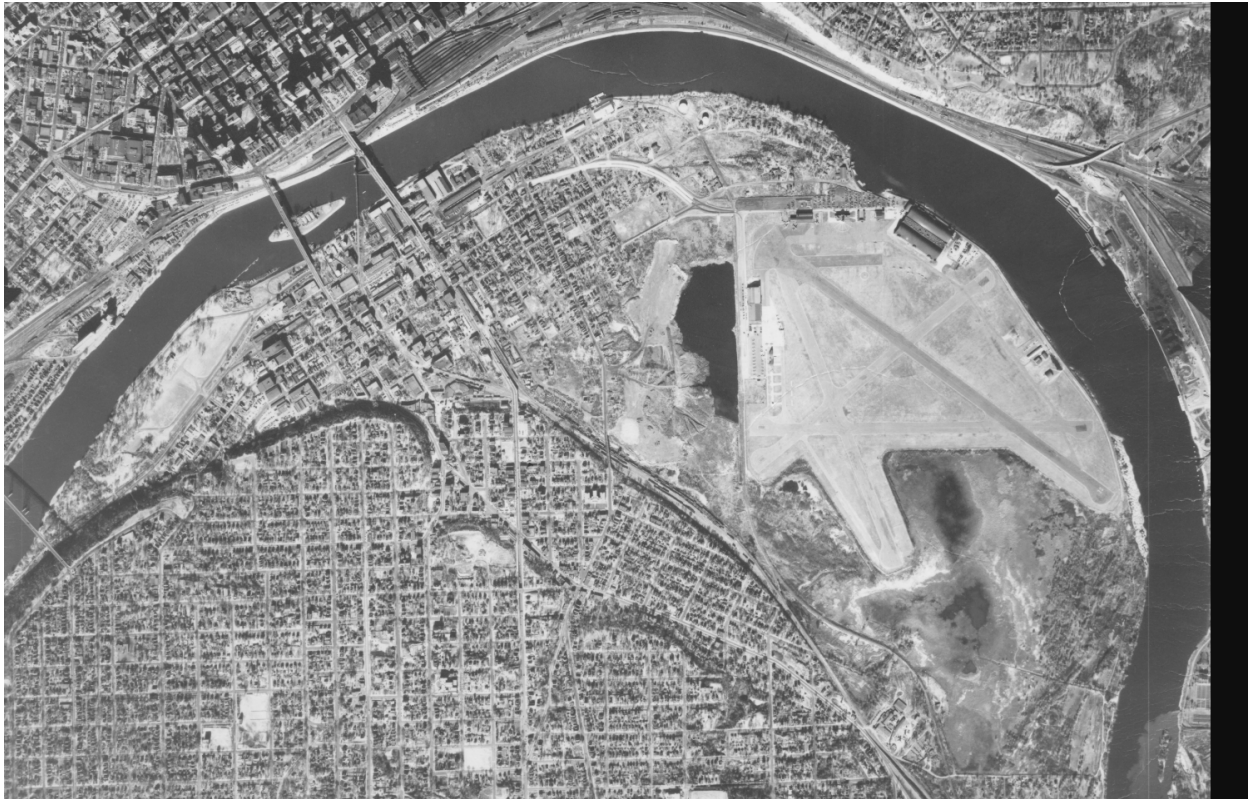
Figure X. Aerial photograph of the West Side, 1953. Photograph courtesy of the Minnesota Historical Aerial Photographs Online, John R. Borchert Map Library, University of Minnesota.
