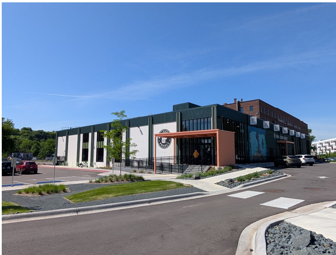
Figure CC. View of north and east elevations of 42 Water Street, looking southwest, June 2026.
