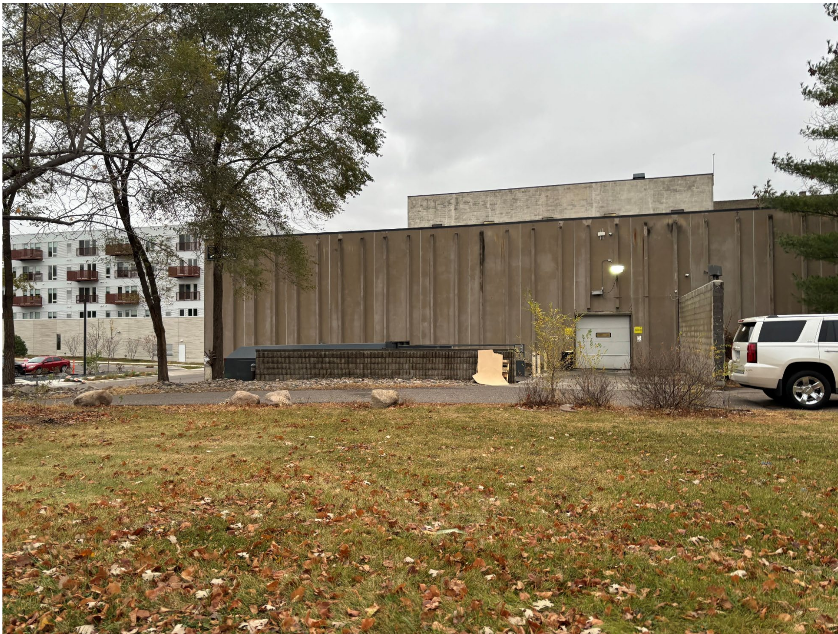
MN_Ramsey County_Farwell, Ozmun, Kirk & Company Warehouses_0007 View of south elevation of Warehouse 3, looking north.
