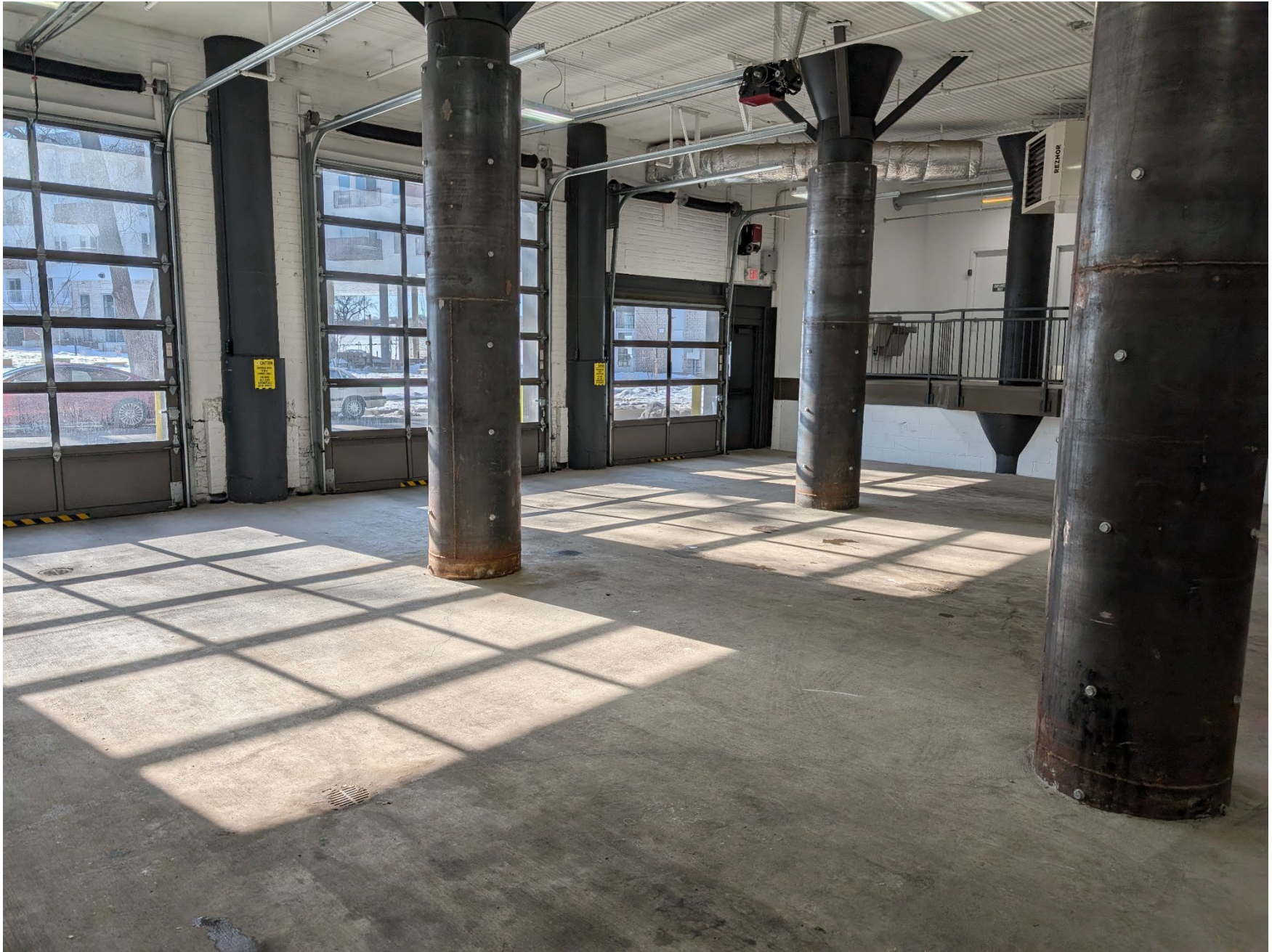
MN_Ramsey County_Farwell, Ozmun, Kirk & Company Warehouses_0016 View of the first level at Warehouse 2, looking northwest.
