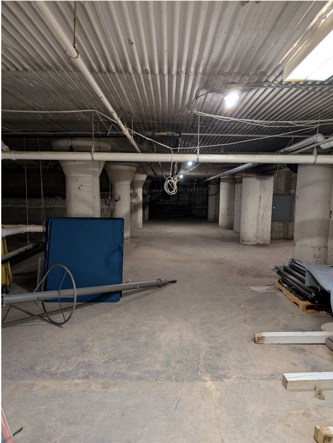
MN_Ramsey County_Farwell, Ozmun, Kirk & Company Warehouses_0014
