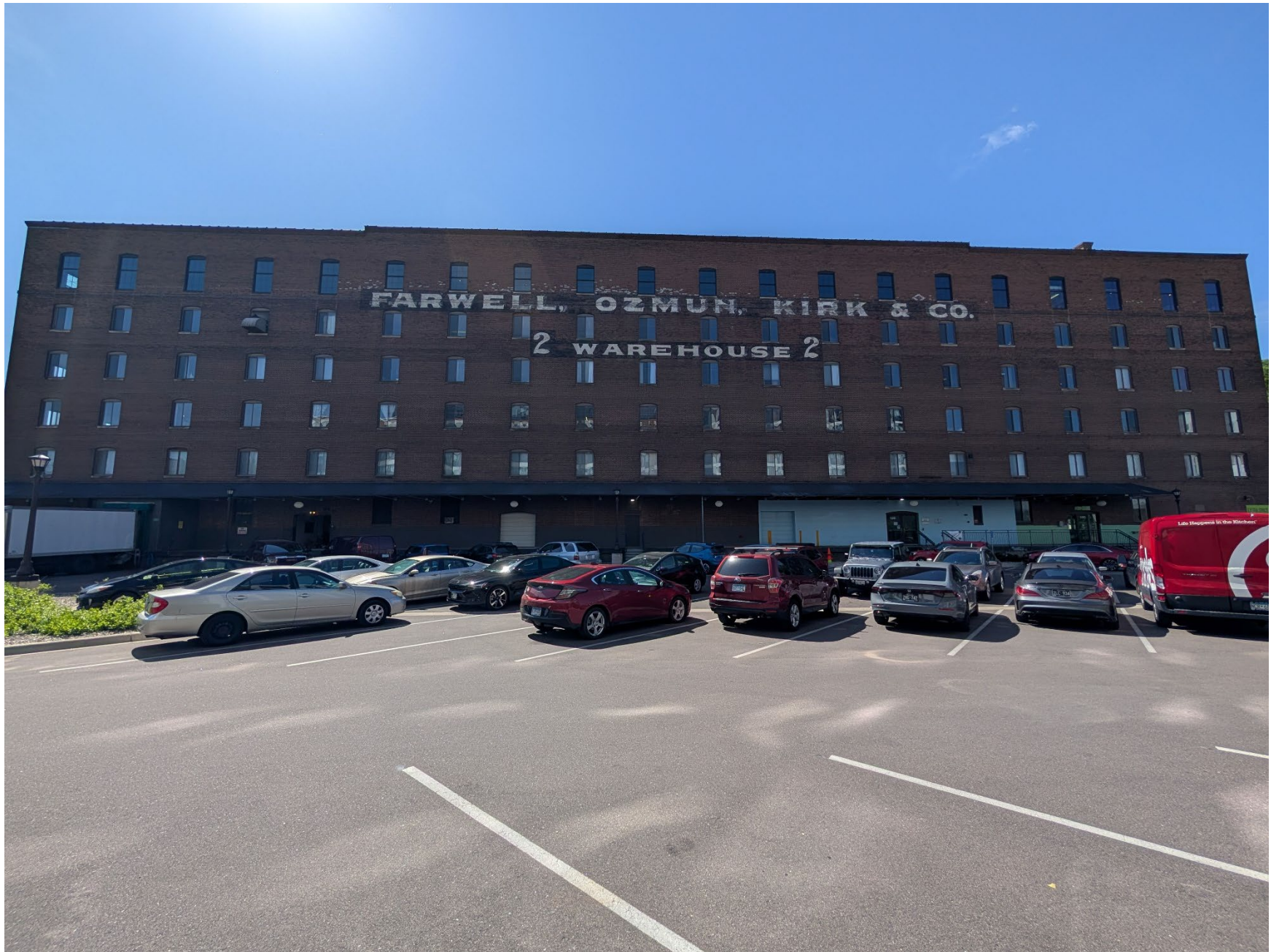
MN_Ramsey County_Farwell, Ozmun, Kirk & Company Warehouses_0001
