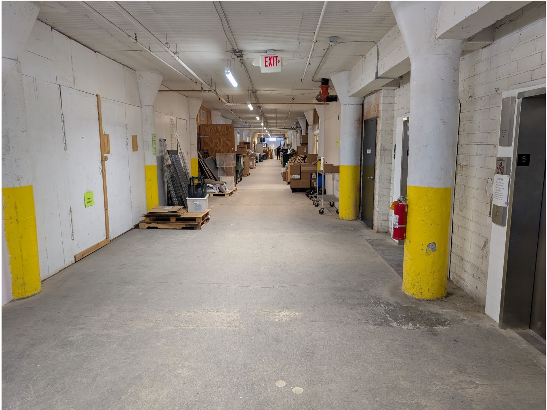
MN_Ramsey County_Farwell, Ozmun, Kirk & Company Warehouses_0022 View of the fifth level at Warehouse 2, looking east.
