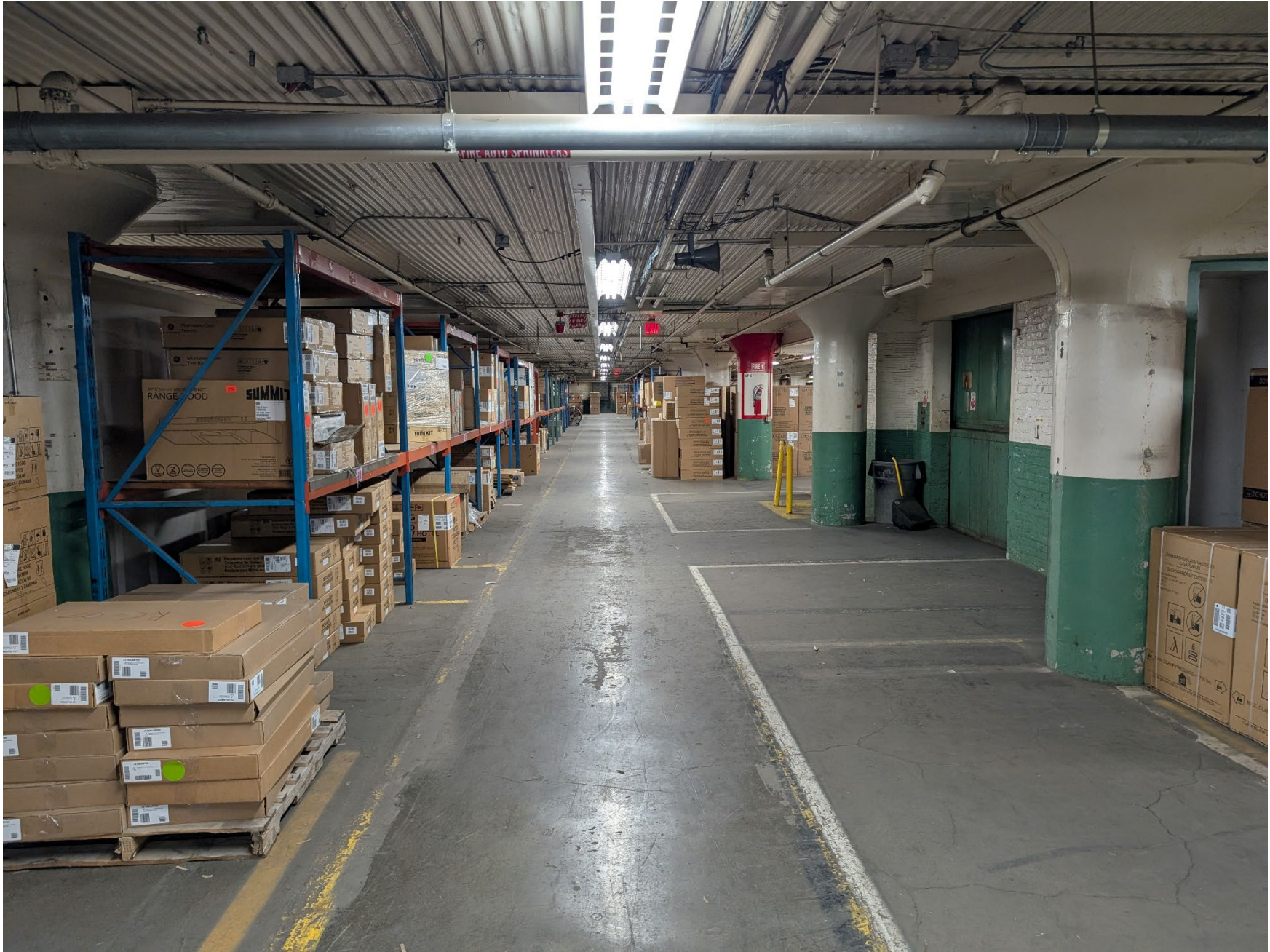
MN_Ramsey County_Farwell, Ozmun, Kirk & Company Warehouses_0028 View of the second level at Warehouse 3, looking west.
