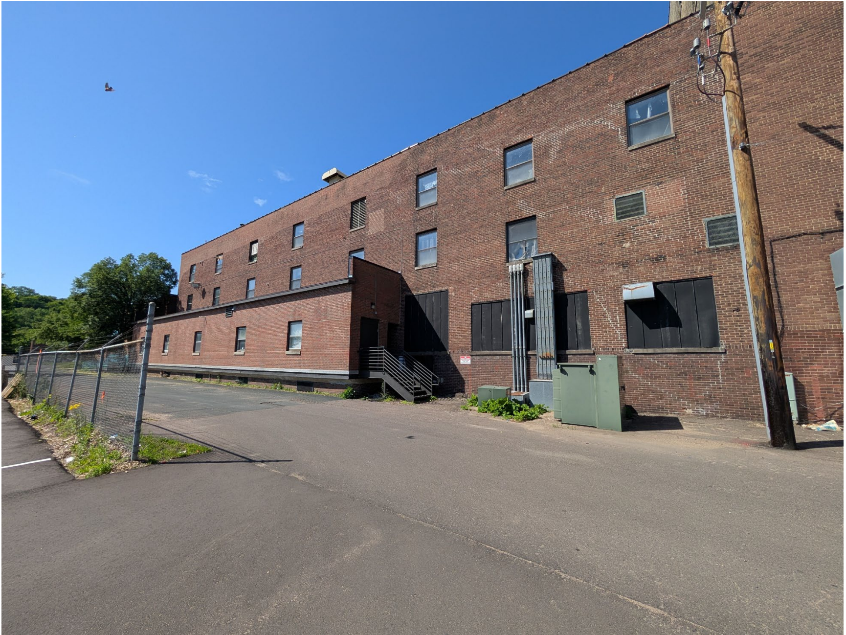
MN_Ramsey County_Farwell, Ozmun, Kirk & Company Warehouses_0012 View of east elevation of Warehouse 3, looking southwest.
