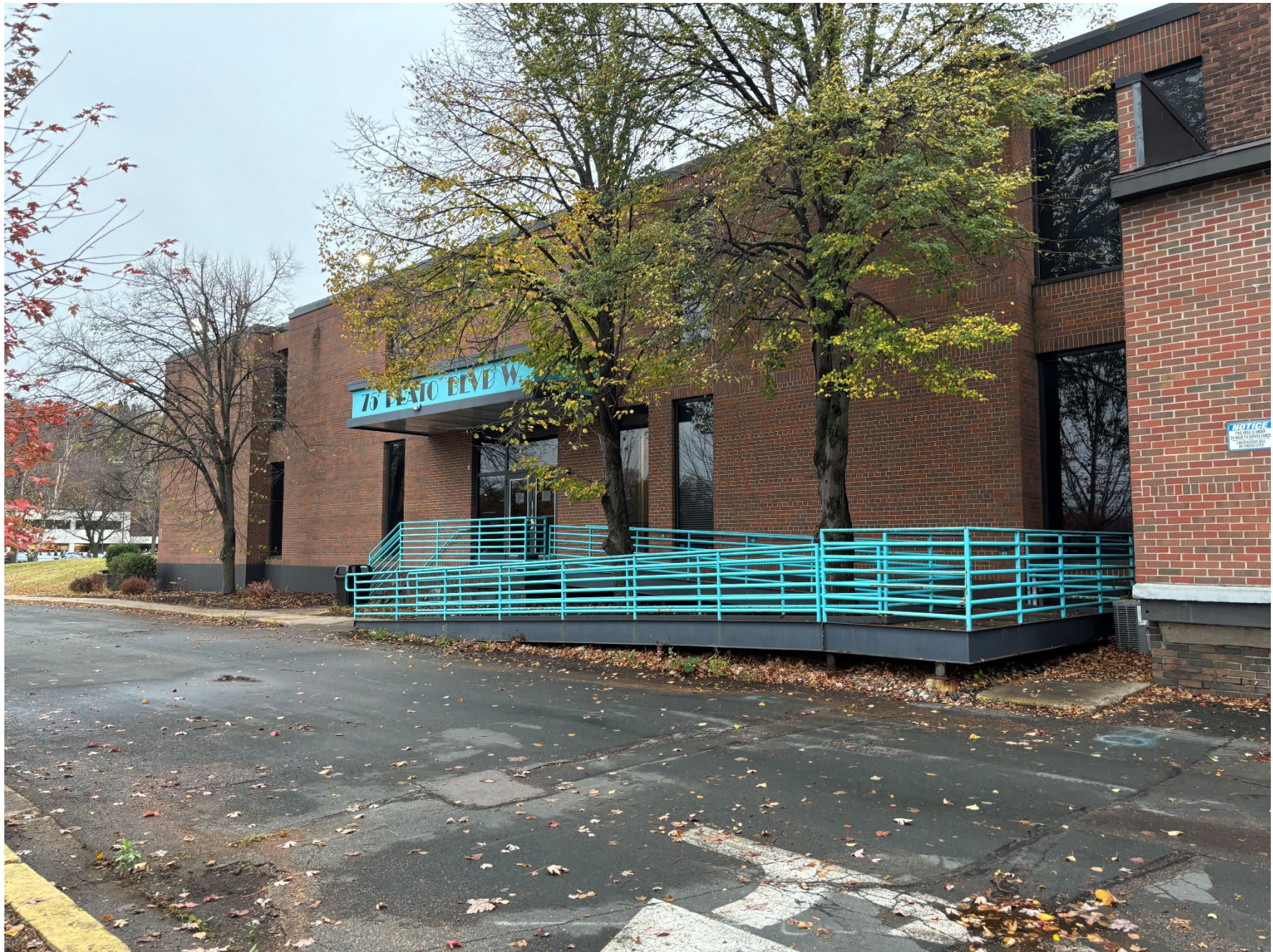
MN_Ramsey County_Farwell, Ozmun, Kirk & Company Warehouses_0010 View of east elevation of Warehouse 3, looking southwest.
