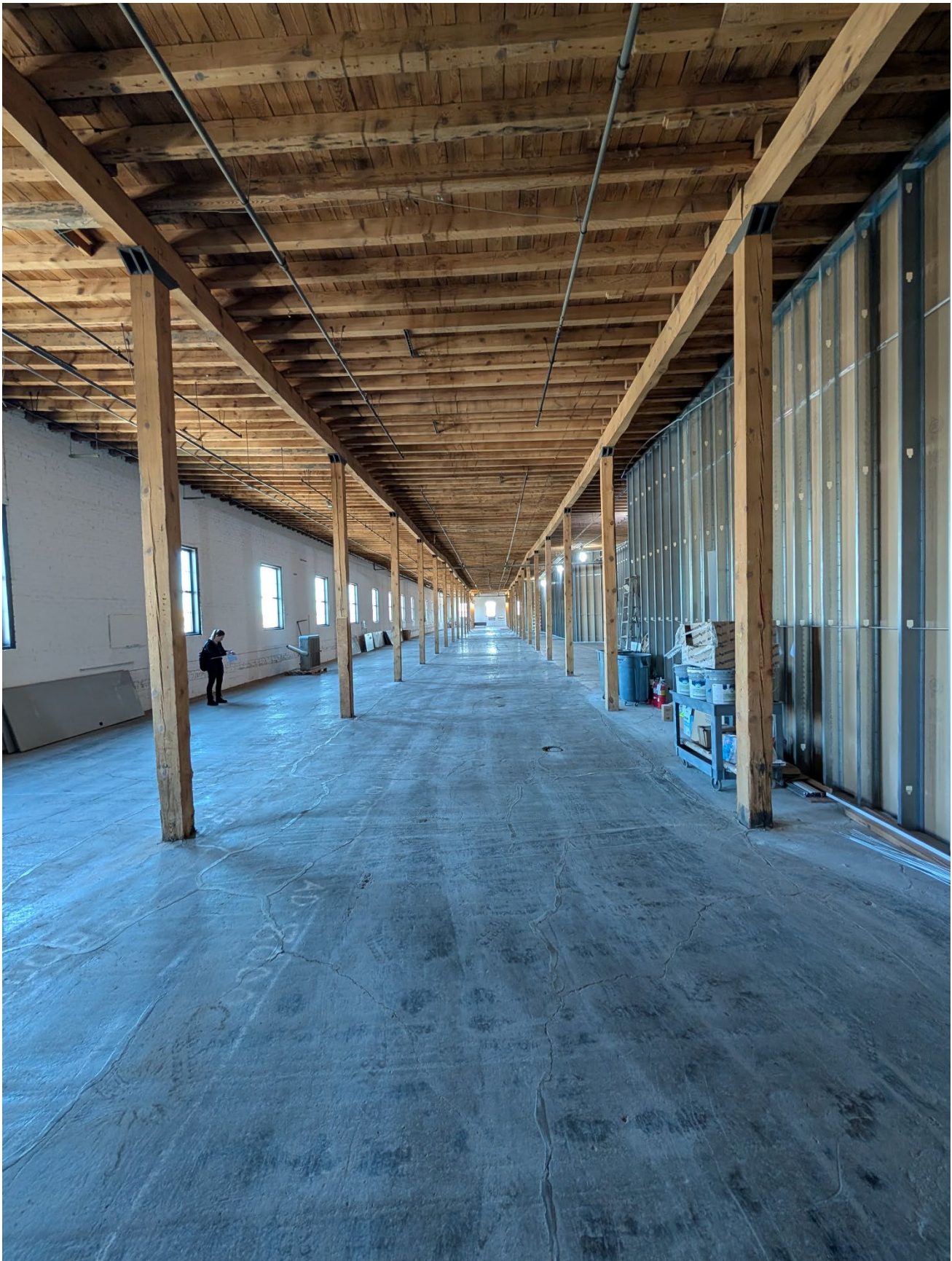
MN_Ramsey County_Farwell, Ozmun, Kirk & Company Warehouses_0024 View of the sixth level at Warehouse 2, looking east.
