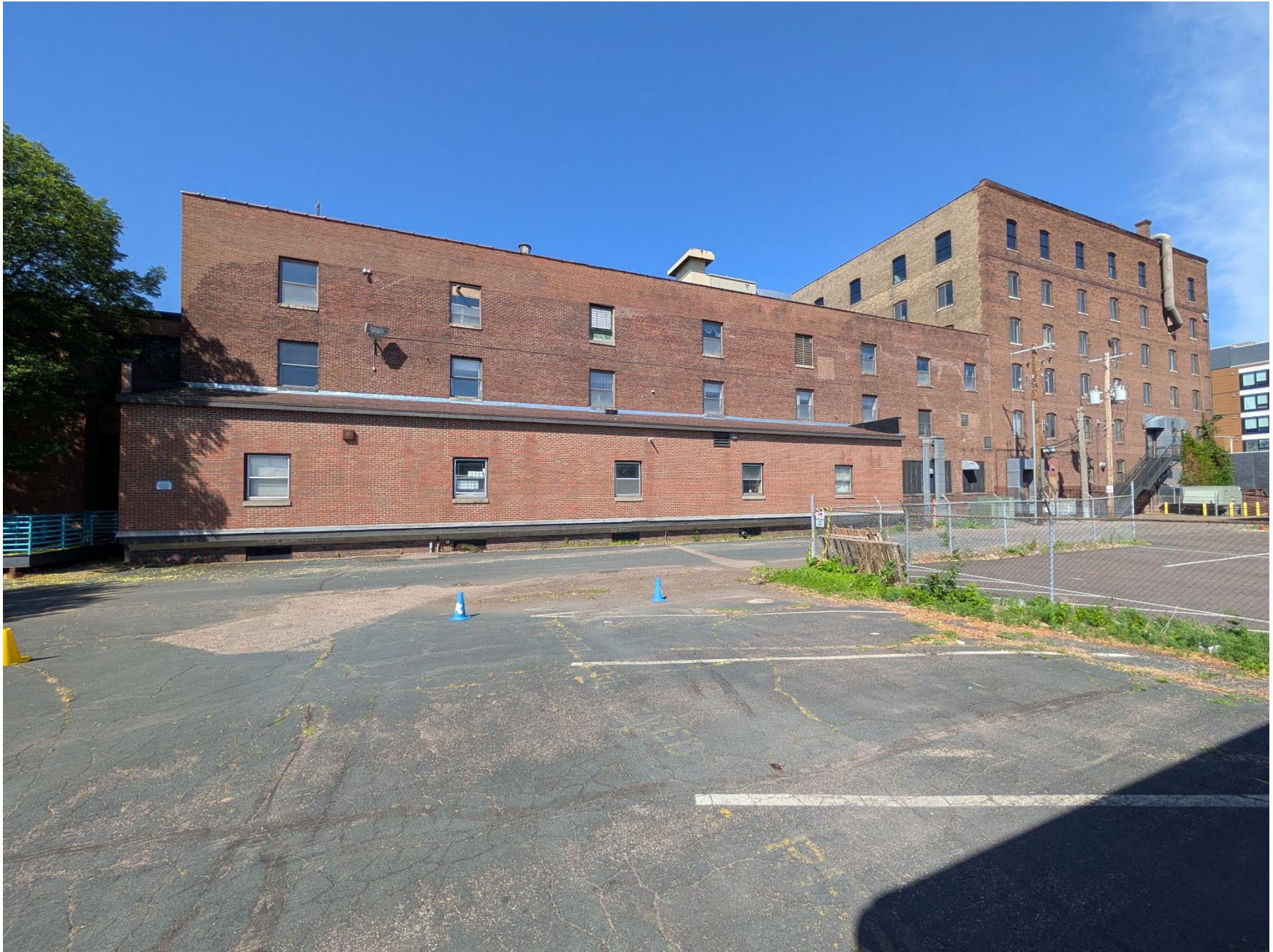
MN_Ramsey County_Farwell, Ozmun, Kirk & Company Warehouses_0011 View of east elevation of Warehouses 2 and 3, looking northwest.
