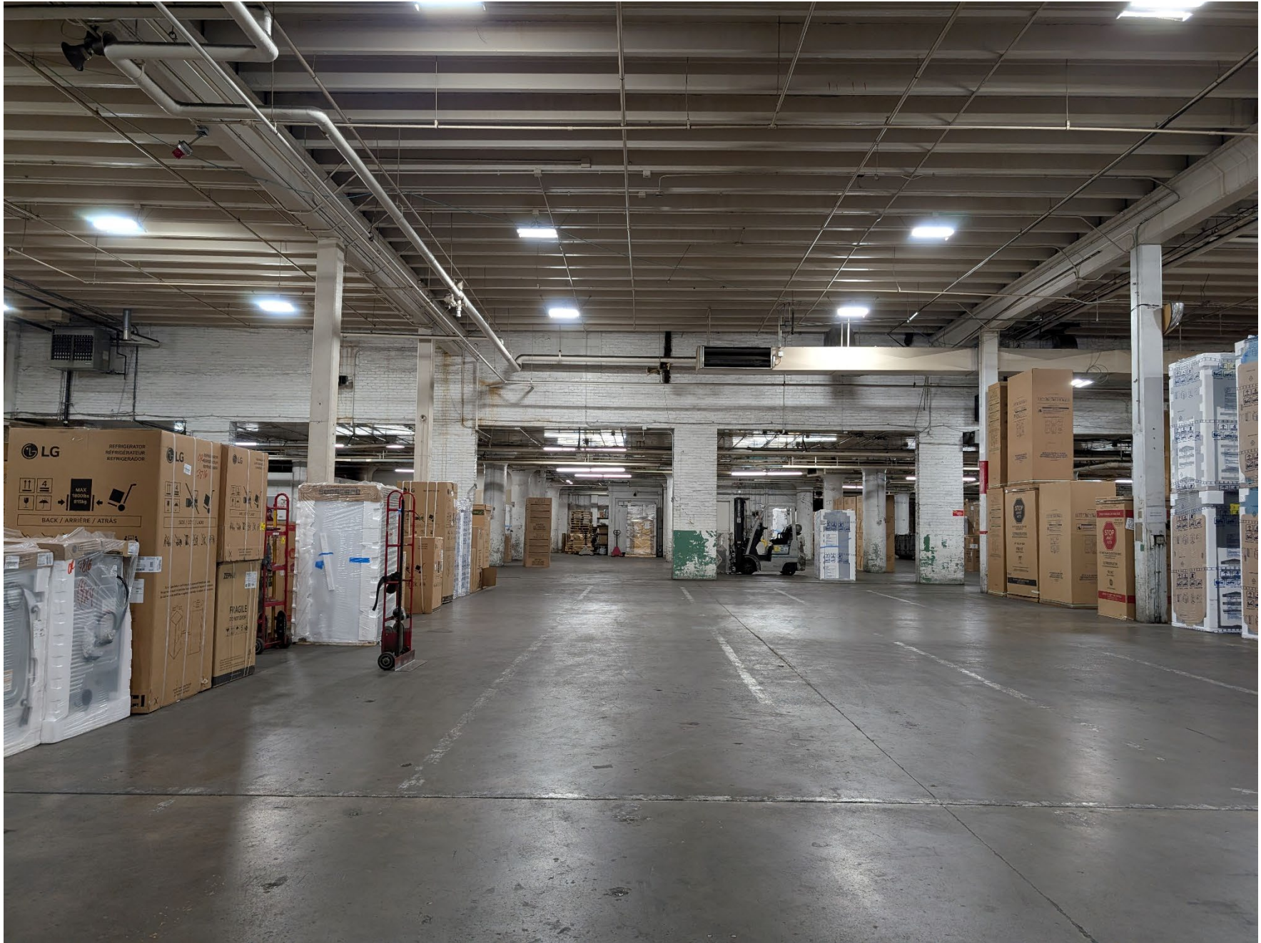
MN_Ramsey County_Farwell, Ozmun, Kirk & Company Warehouses_0027 View of the first level at Warehouse 3, looking north.
