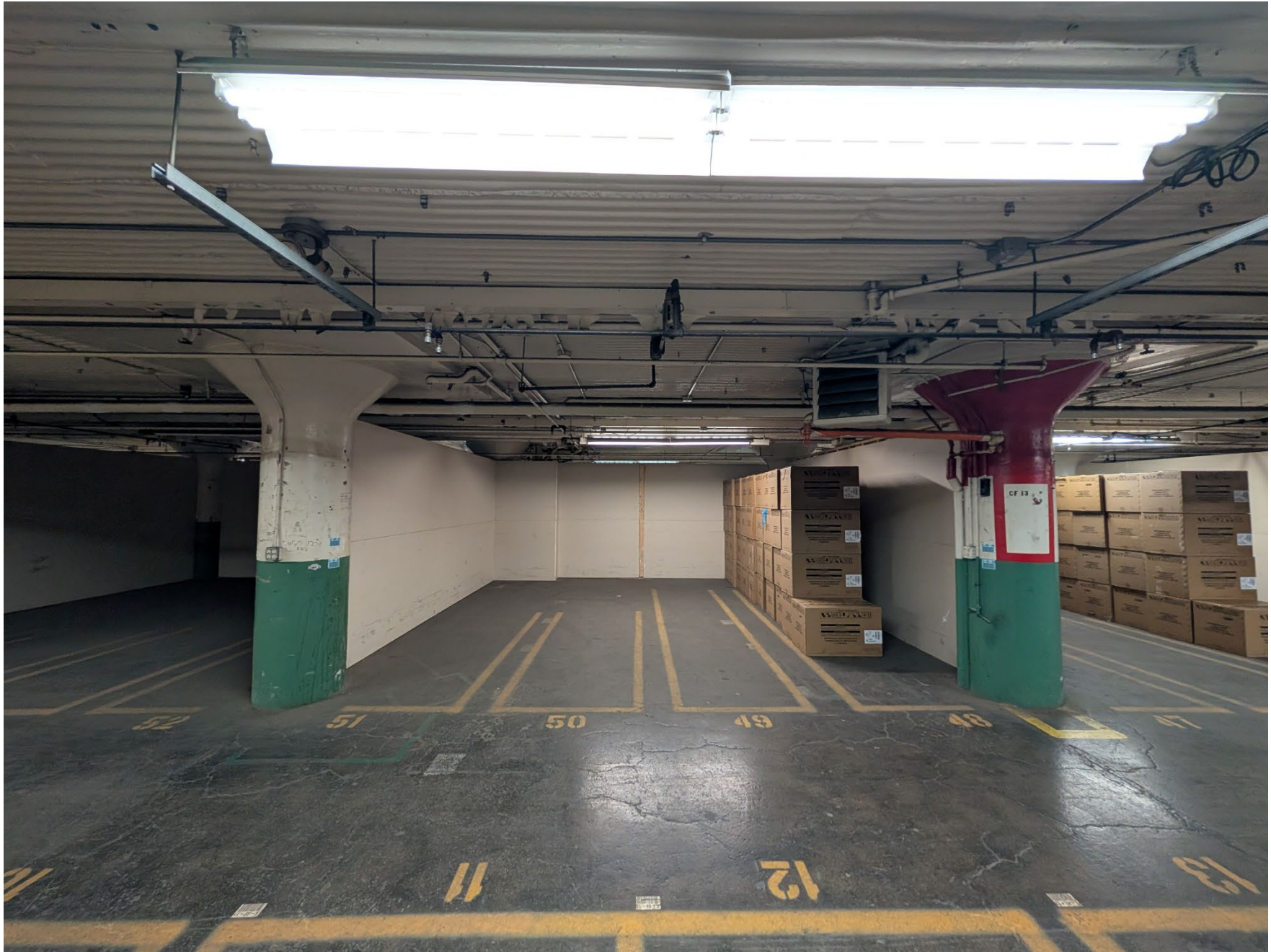
MN_Ramsey County_Farwell, Ozmun, Kirk & Company Warehouses_0029 View of the second level at Warehouse 3, looking north.
