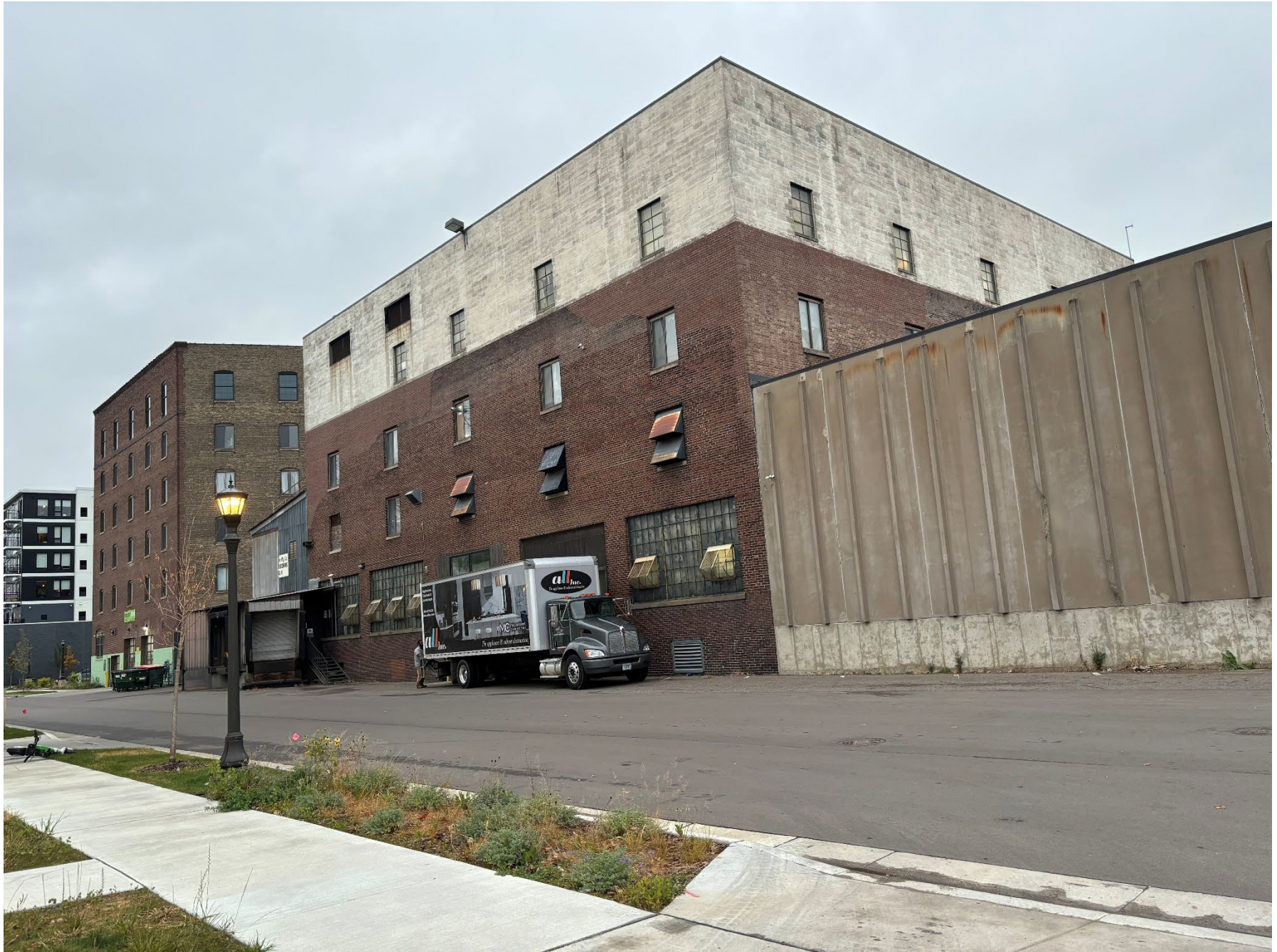
MN_Ramsey County_Farwell, Ozmun, Kirk & Company Warehouses_0005 View of west elevation of Warehouse 3, looking northeast.
