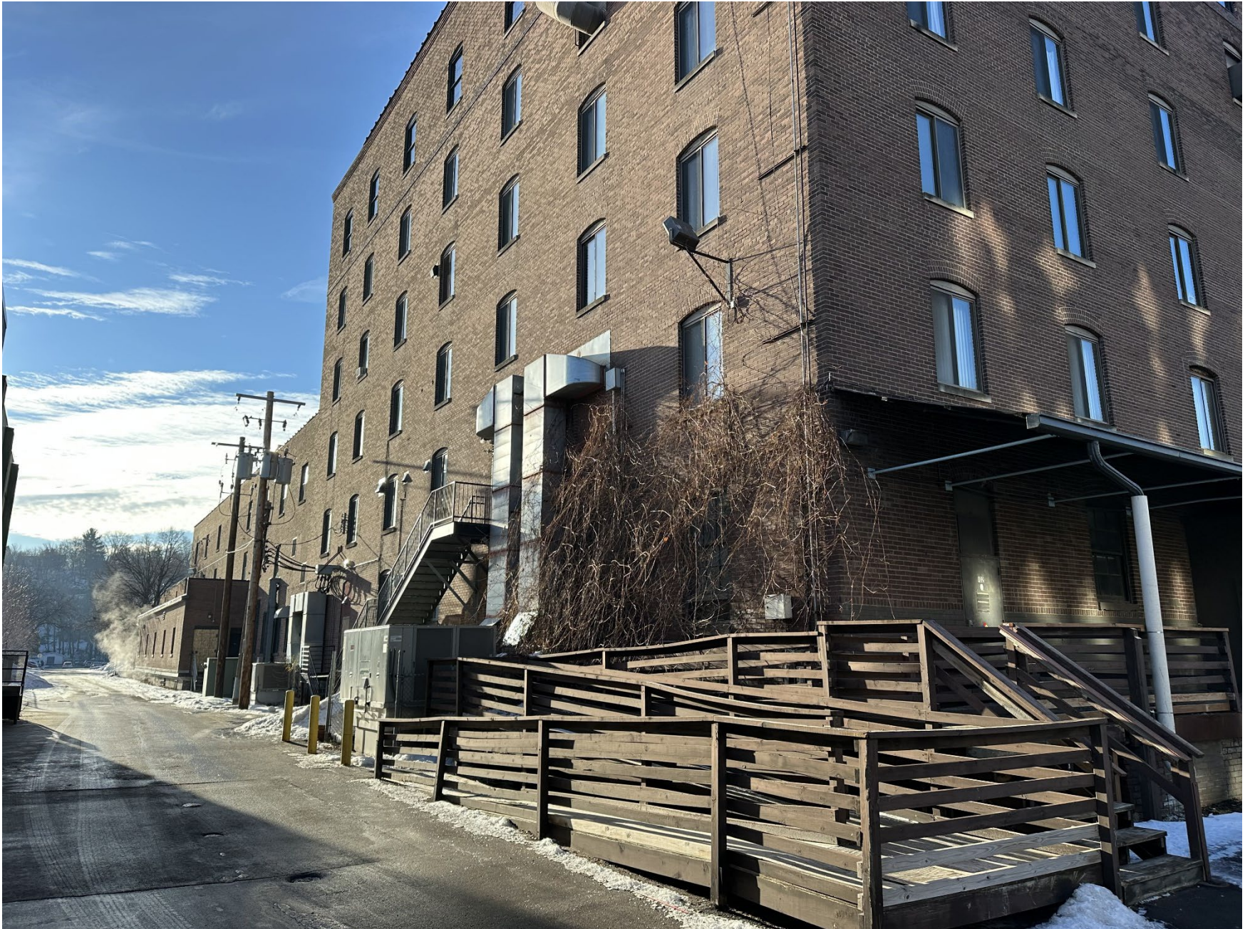
MN_Ramsey County_Farwell, Ozmun, Kirk & Company Warehouses_0013
