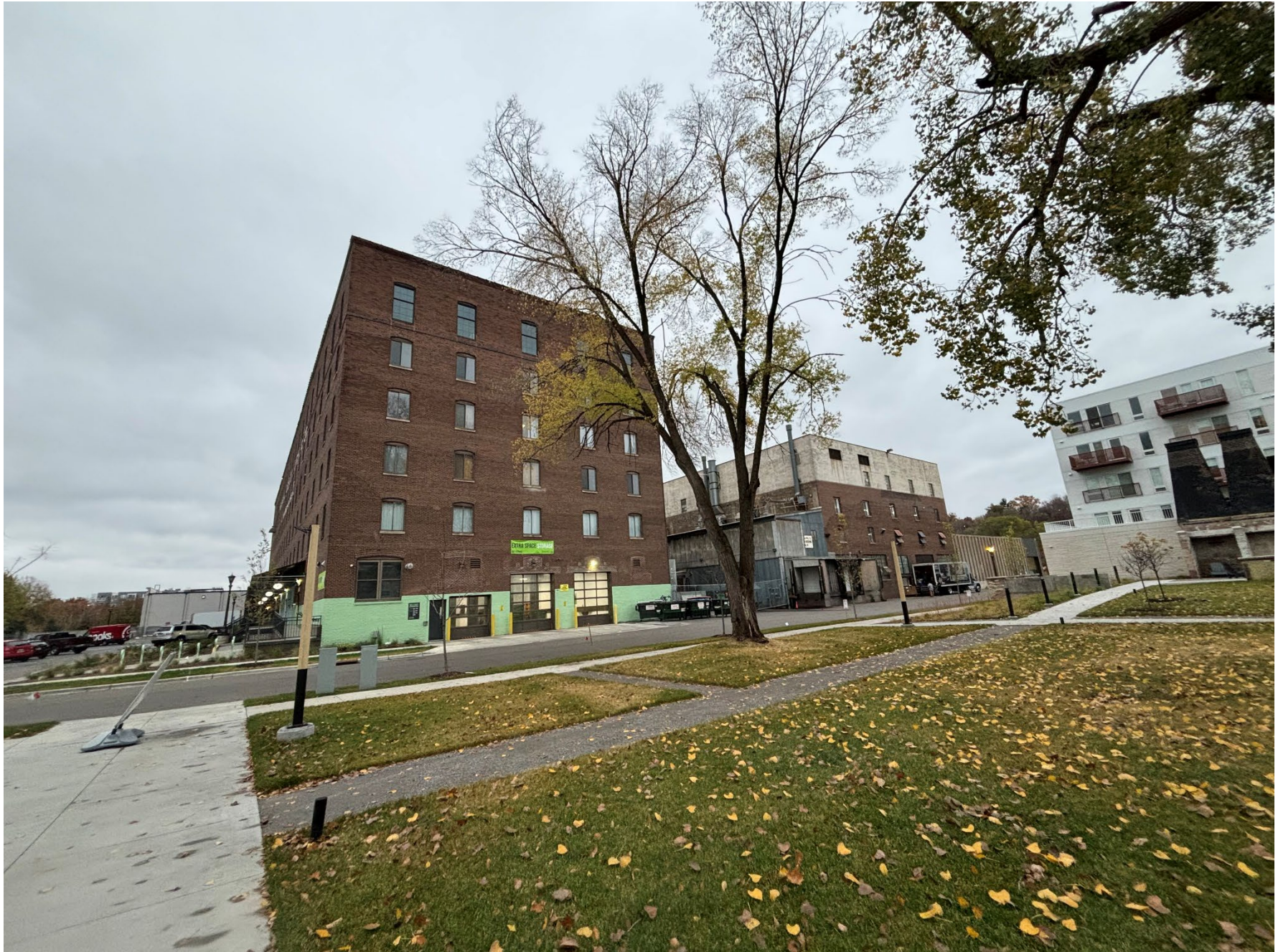
MN_Ramsey County_Farwell, Ozmun, Kirk & Company Warehouses_0003 View of west elevations of Warehouses 2 and 3, looking southeast.
