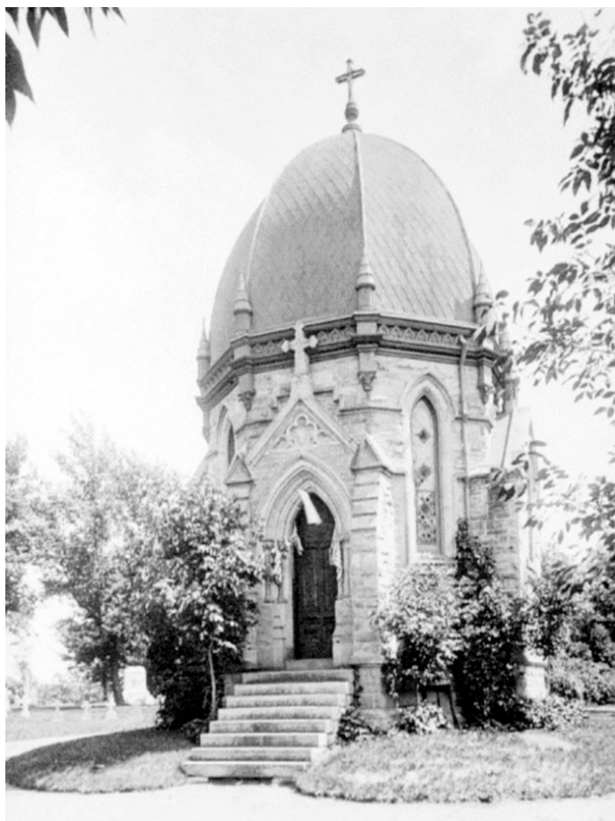
Figure 4: ca.1906, Cemetery Chapel. (Image courtesy of the Archdiocese of Saint Paul and Minneapolis). The cemetery chapel first appears on the 1884 plat map, Block 7. This image documents the building in 1906, revealing it as a stone structure with a hexagonal, domed roof, and a design character that reflects the influence of medieval precedents, including the use of buttresses and Gothic arched openings. Historic aerial photographs indicate the building was extant through 1957. The Archdiocese does not have a record of its demolition - neither the reason for its removal nor the year undertaken.
