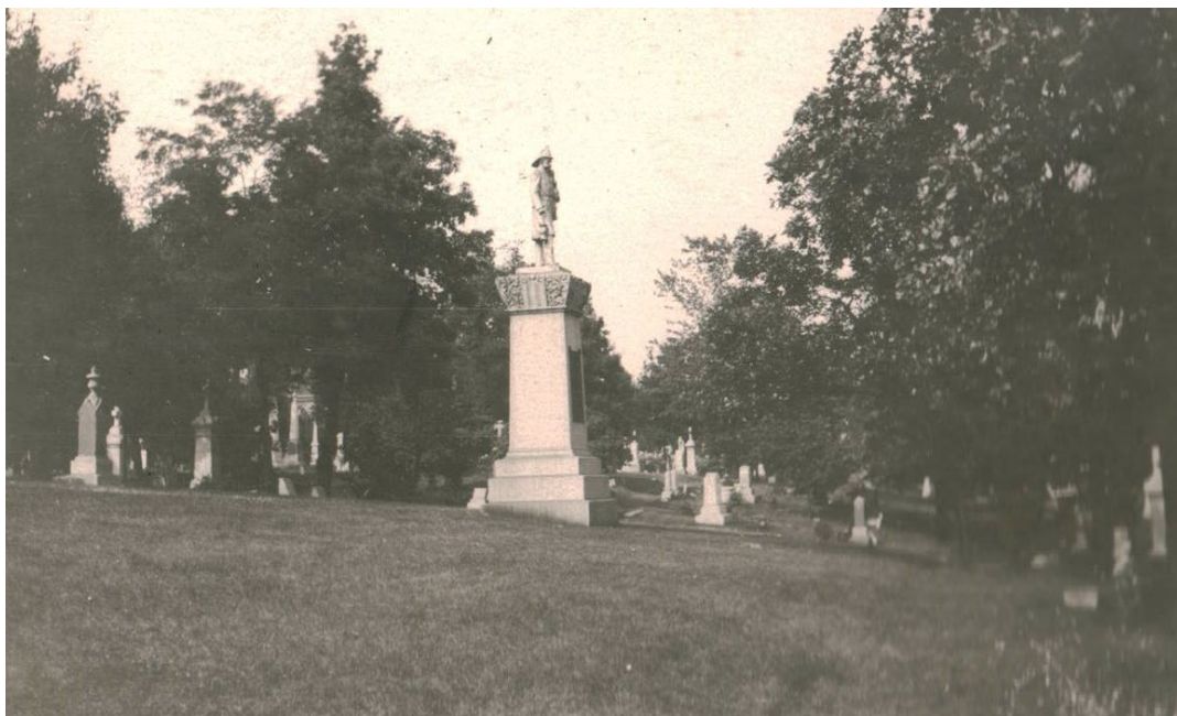
Figure 9: ca.1906, Cemetery View with the Firefighters Monument (Original Section, Block 5), looking NE. (Image courtesy of the Archdiocese of Saint Paul and Minneapolis).
