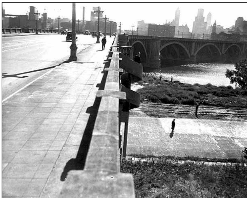
Figure 7. Third Avenue Bridge at north approach span, ca. 1935 ( Minnesota Historical Society )
