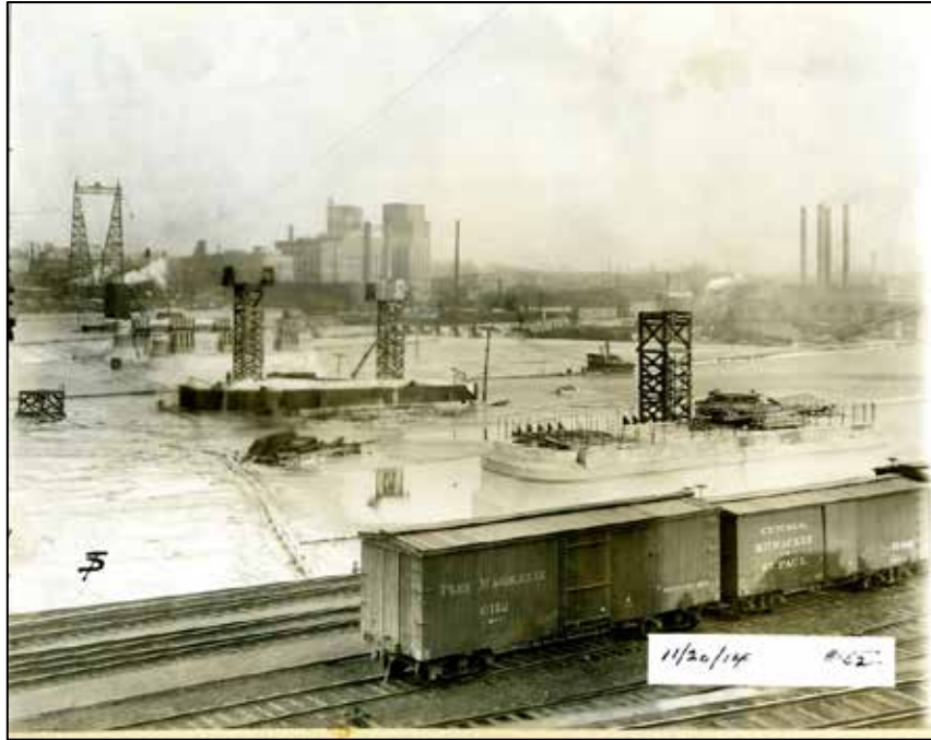
Figure 1. November 20, 1914 – Construction of piers, looking northeast ( City of Minneapolis )
