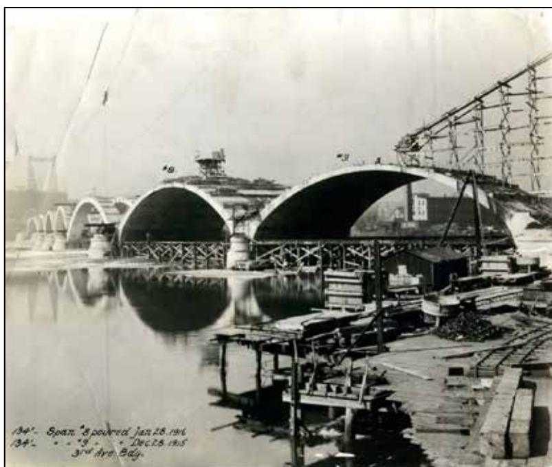
Figure 4. c. 1916 – Arch construction, looking west ( City of Minneapolis )
