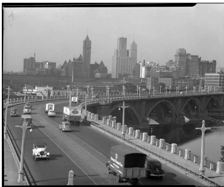
Figure 10. Third Avenue Bridge, ca. 1958 ( Minnesota Historical Society )
