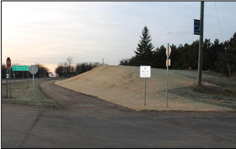
Damaged area of 21OT13 after restoration.
