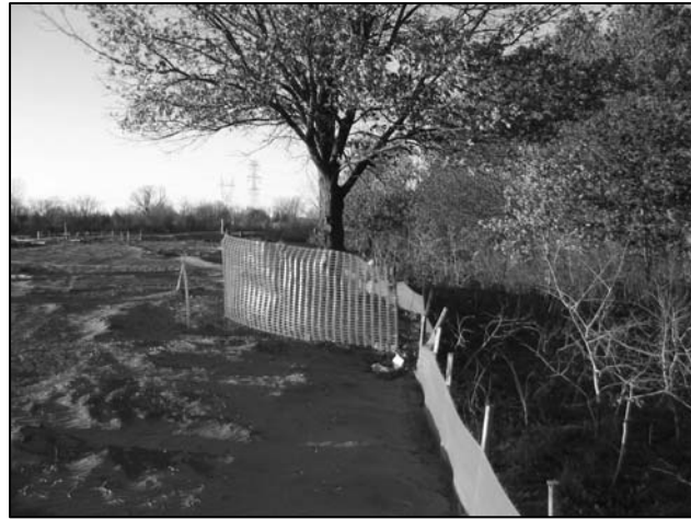
Mound (beneath tree) protected by fence within construction area at Savage Lofts project.
